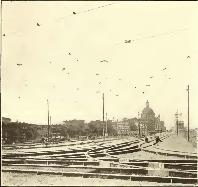
FIG. 6.—OVERHEAD CONSTRUCTION ON BROOKLYN PLAZA
