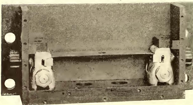
FUSE BOX AND FUSE
