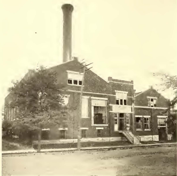
THE NEW POWER HOUSE OF THE LIMA ELECTRIC RAILWAY & LIGHT COMPANY
