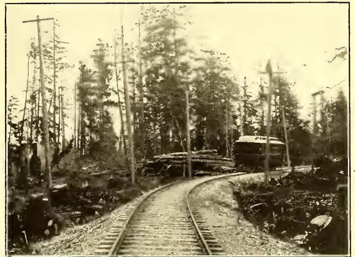
A VIEW ON THE LINE OF THE GRAY'S HARBOR ELECTRIC COMPANY, NEAR ABERDEEN
