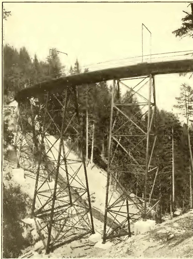
HIGH STEEL VIADUCT NEAR KREIT-STUBAITHALBAHN
