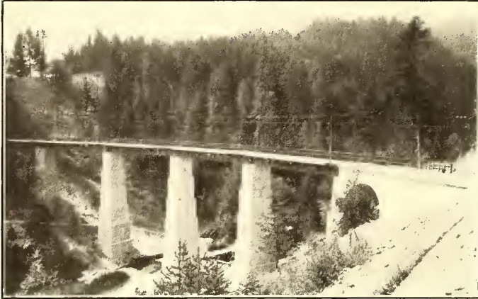
BRIDGE ON CONCRETE PIERS—STUBAITHALBAHN
