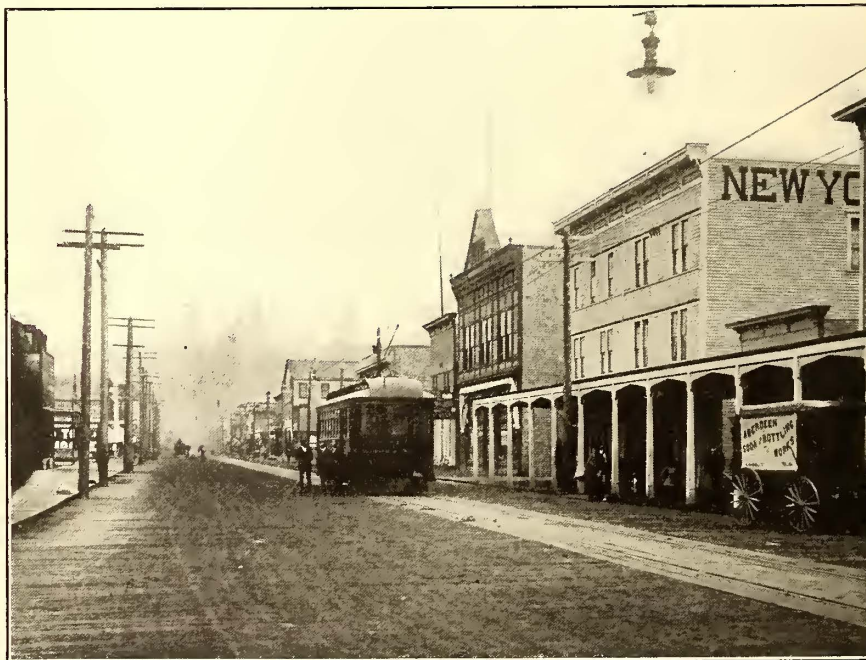
PLANKED ROADWAY ON EIGHTH STREET, HOQUIAM
