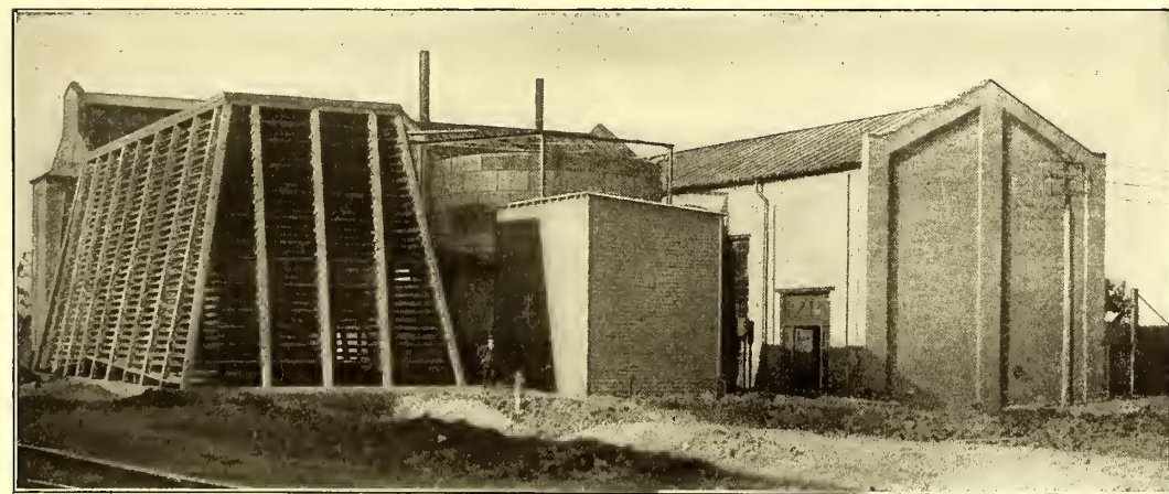
GENERAL VIEW OF POWER PLANT, SHOWING COOLING TOWER AND GAS TANKS
