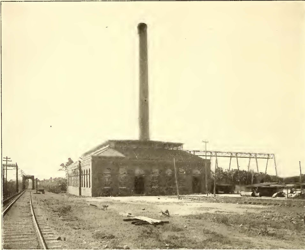
EXTERIOR OF POWER STATION
