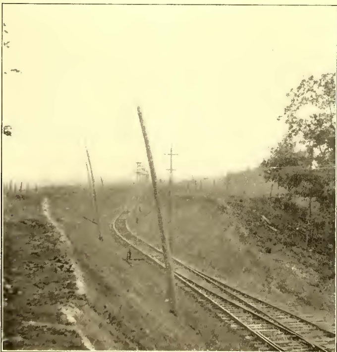
CUT NEAR RIDGE POINT PARK
