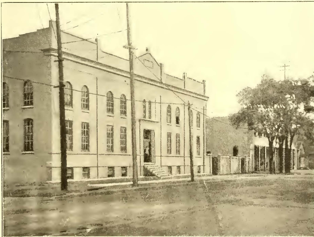
POWER HOUSE, CAR HOUSE AND OFFICES
