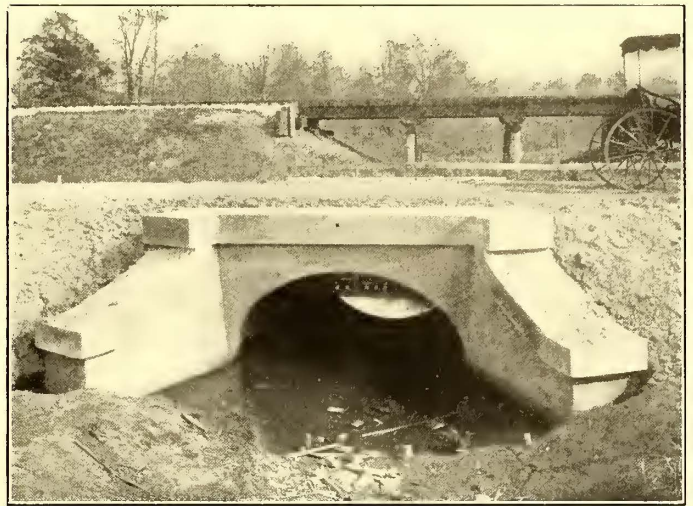
TYPICAL CONCRETE ARCH BRIDGE
