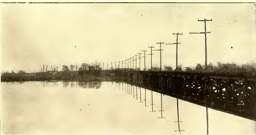
2810-FT. TRESTLE OVER THE FILTER BEDS OF THE BOX BOARD WORKS NEAR NOBLESVILLE
