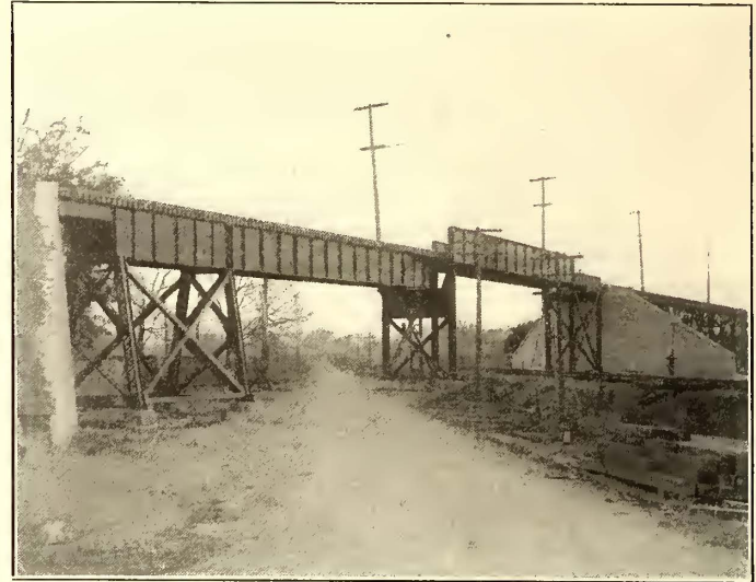
CROSSING OF THE LAKE ERIE & WESTERN NEAR NOBLESVILLE
