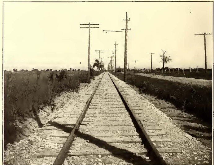
STANDARD ROADBED AND OVERHEAD CONSTRUCTION BETWEEN JOLIET AND PLAINFIELD
