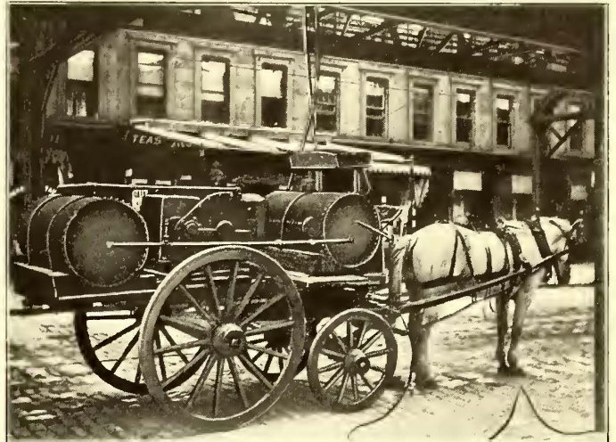
FIG. 3.—PORTABLE SAND-BLAST OUTFIT
