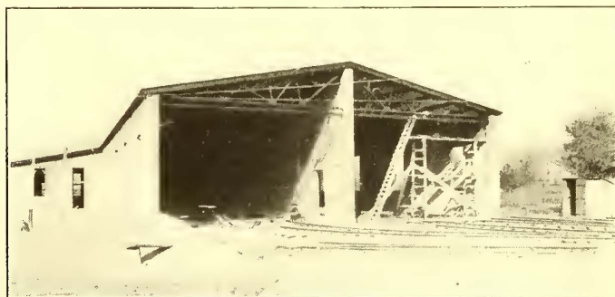
CAR SHOP AND STORAGE IN COURSE OF ERECTION AT PLAINFIELD
