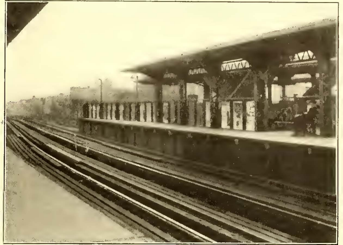
CONCRETE STATION PLATFORM AND ROOF, METROPOLITAN ELEVATED RAILWAY, CHICAGO
