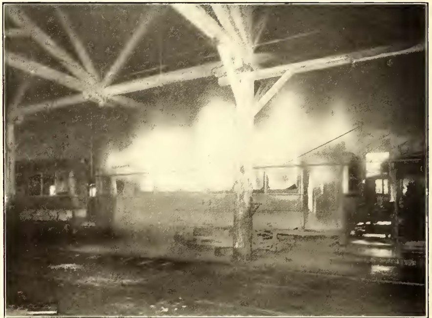
CAR IN TEST NO. 3—DURING THE FIRE
