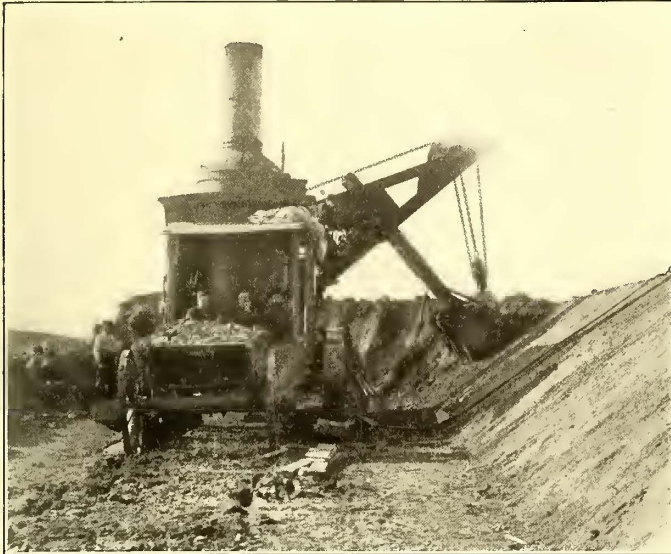
VIEW SHOWING THE FINE SLOPE GIVEN BY STEAM SHOVEL
