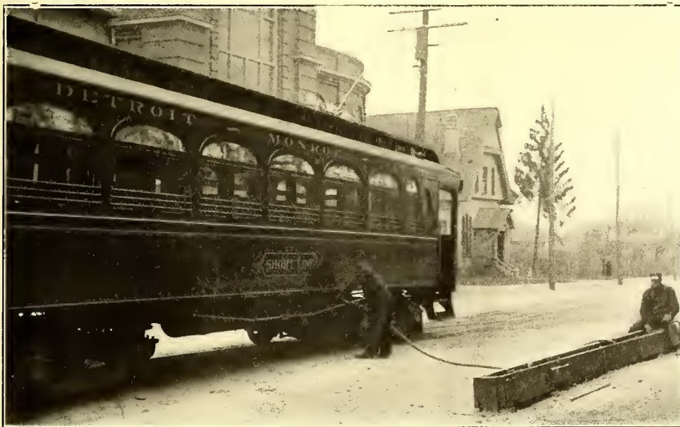
VIEW OF CAR AT THE STORAGE-AIR SYSTEM STATION AT THE MAIN POWER STATION IN MONROE, SHOWING METHOD OF CHARGING THE CAR RESERVOIRS WITH THE HIGH-PRESSURE AIR
