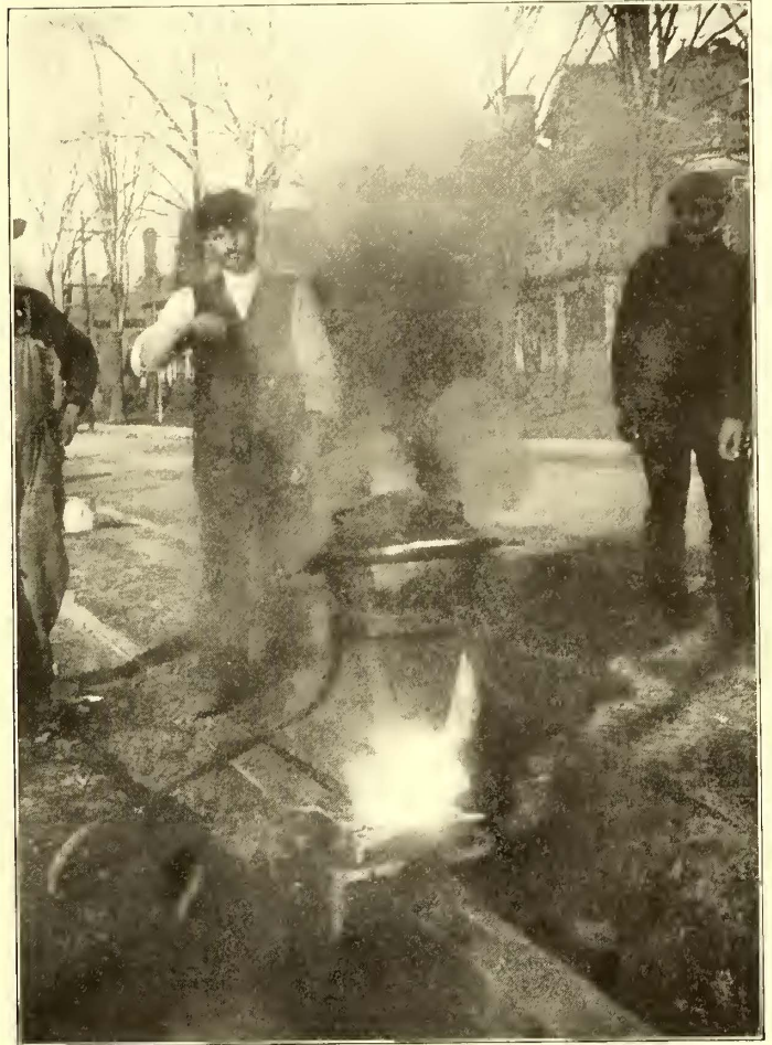
DURING THE POUR, SHOWING THE MOLTED METAL FLOWING INTO MOULD
