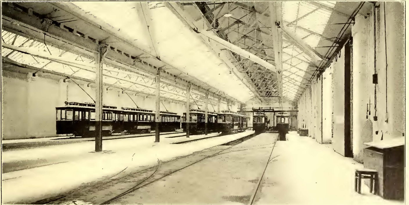
SIX-TRACK CAR SHED OF THE HONG KONG TRAMWAYS, 220 FT. LONG, AND ACCOMMODATING THIRTY-FIVE 29-FT. CARS
