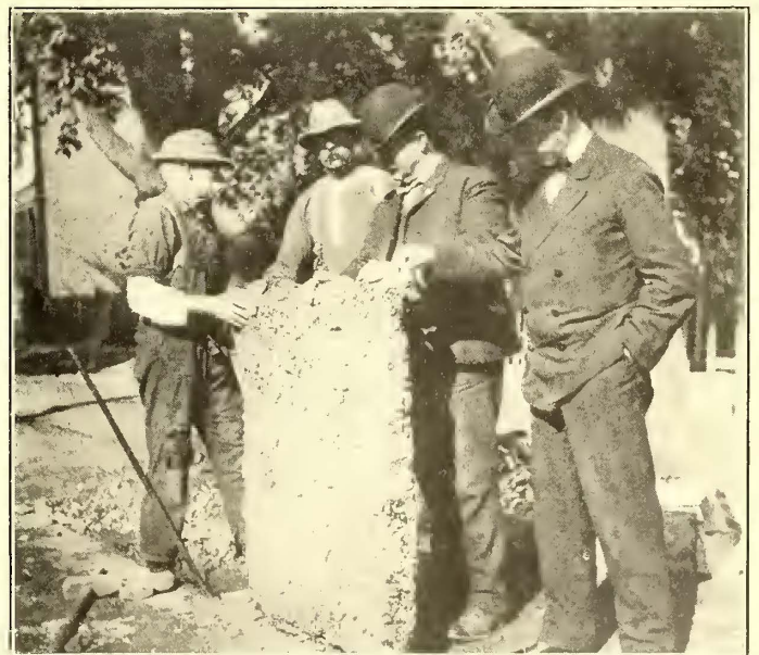
BOSTON ELEVATED RAILWAY, HIGH STREET, MEDFORD, SHOWING TIE THICKNESS AND UNDER SIDE OF A SECTION OF THE BITULITHIC PAVEMENT, CUT FROM BETWEEN THE TRACKS TO INSTALL A CATCH-BASIN INLET
