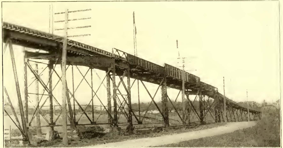
FIG. 24.—ANOTHER VIEW OF THE VIADUCT OVER THE VANDALIA RAILROAD, AT GLEN STOCK FARM
