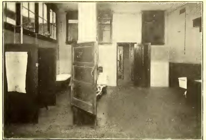
BATHS, SHOWERS AND WASH BOWLS IN THE EMPLOYEES' TOILET ROOMS
