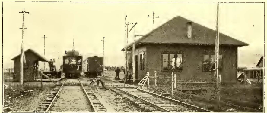
THE GREEN ACRES SUB-STATION OF THE COEUR D'ALENE & SPOKANE RAILWAY
