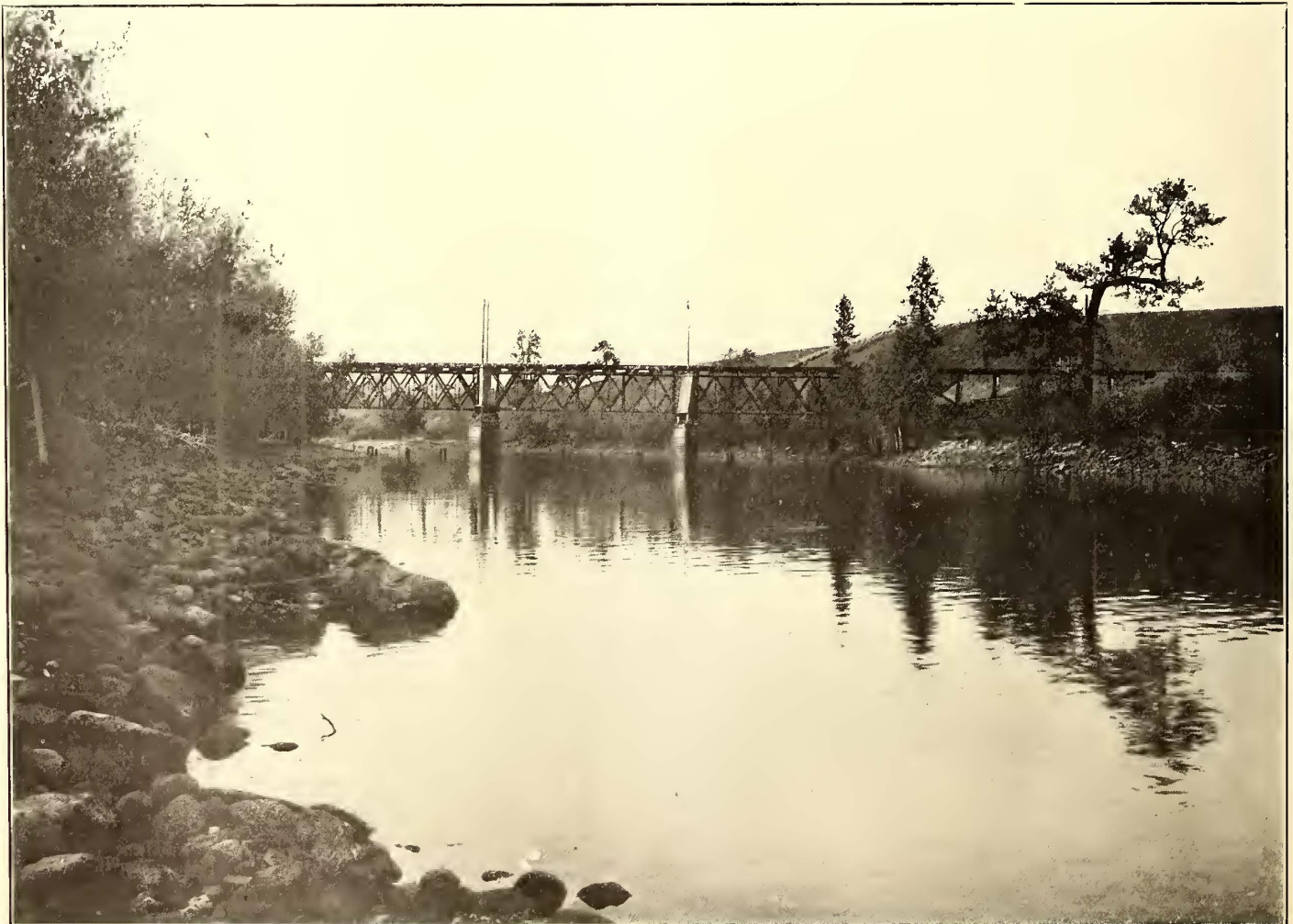
BRIDGE CROSSING SPOKANE RIVER; ALSO SHOWING THE IDAHO-WASHINGTON BOUNDARY LINE
