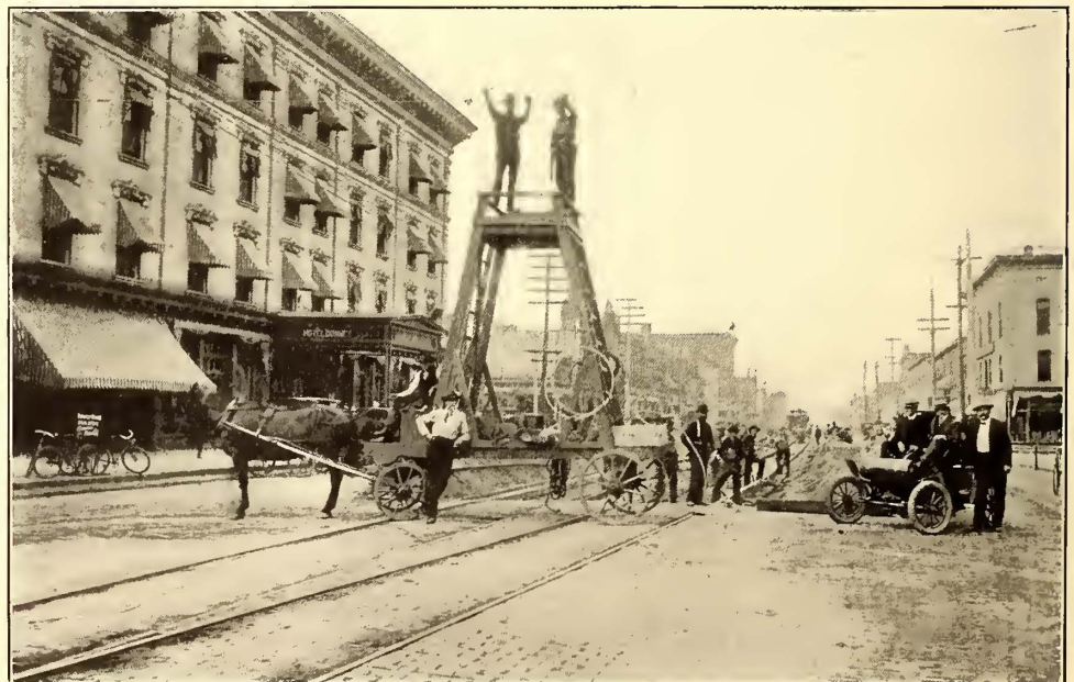
OVERHEAD LINE AND TRACK CONSTRUCTION VIEW IN THE CITY OF LANSING
