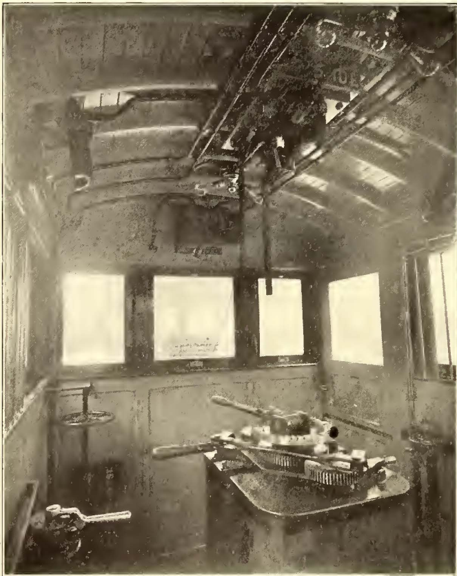
INTERIOR VIEW IN CAB OF THE BROOKLYN ELECTRIC LOCOMOTIVE, SHOWING CONTROL APPARATUS
