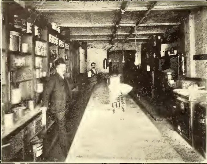
THE FIREPROOF PAINT STOCK AND SUPPLY ROOM FOR USE OF THE PAINT SHOP DEPARTMENT
