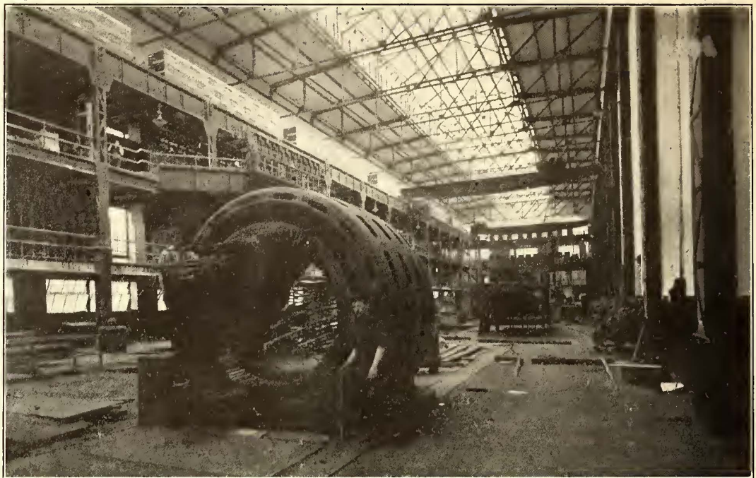
FIG. 28.—ALTERNATOR FIELD DURING ERECTION
