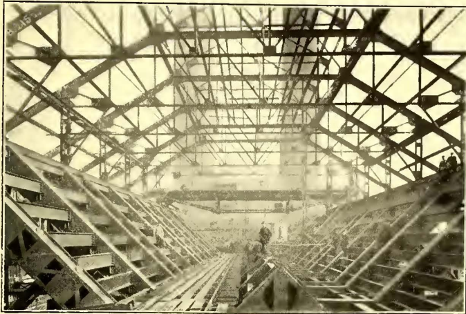
FIG. 20.—COAL BUNKERS IN PROCESS OF ERECTION
