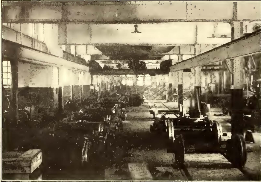
FIG. 8.—GENERAL VIEW OF TRACKS UNDER TRAVELING CRANE
