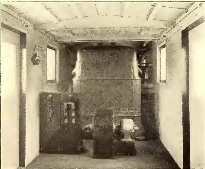
FIG. 2.—INTERIOR VIEW OF CAR, SHOWING TRANSFORMER, BLOWER SET, OIL-SWITCH LEVER AND STARTING PANEL
