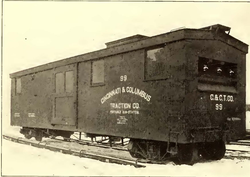
FIG. 1.—EXTERIOR VIEW OF 400-KW PORTABLE SUB-STATION, TRANSMISSION POTENTIAL 16,500 OR 23,000 VOLTS
