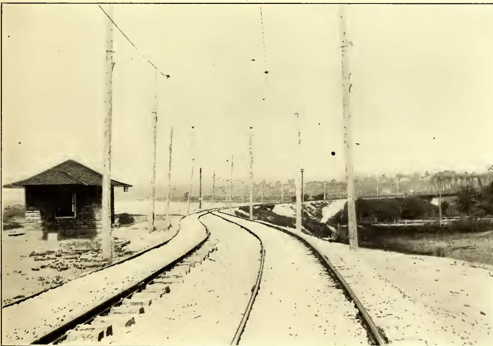
FORT MEIGS STATION, HEAVY FILL APPROACHING MAUMEE RIVER BRIDGE, TOLEDO, BOWLING GREEN & SOUTHERN RAILWAY
