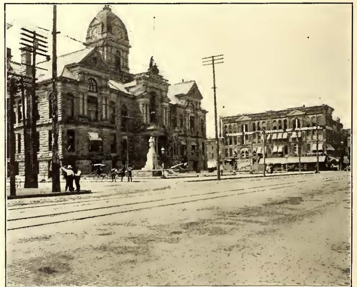
MAIN STREET IN FINDLAY, LAID WITH T-RAIL
