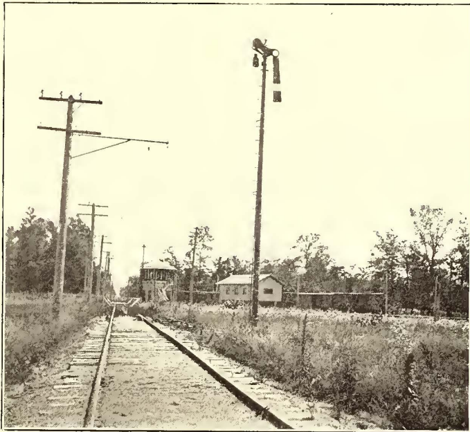
CROSSING OF THE TOLEDO & WESTERN RAILWAY AND THE WABASH RAILROAD, SHOWING INTERLOCKER, TRANSFER TRACKS AND TRANSFER STATION
