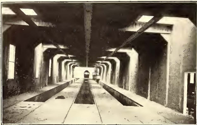
FIG. 5.—INTERIOR OF COMPLETED CONCRETE CAR HOUSE
