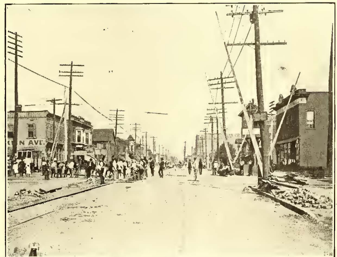
ST. CLAIR AVENUE, LOOKING WEST
