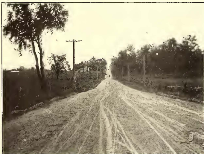
SOME LONG GRADES, SHOWING REPAIR WORK DONE BY THE COMPANY
