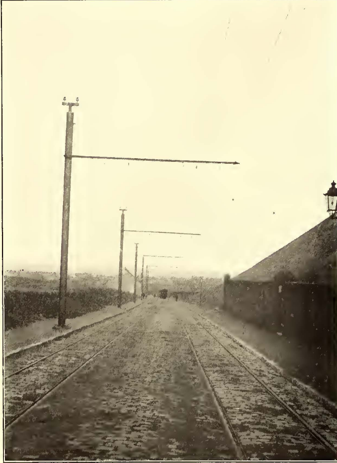
DOUBLE-TRACK SECTION ON THE BORINAGE SINGLE-PHASE RAILWAY
