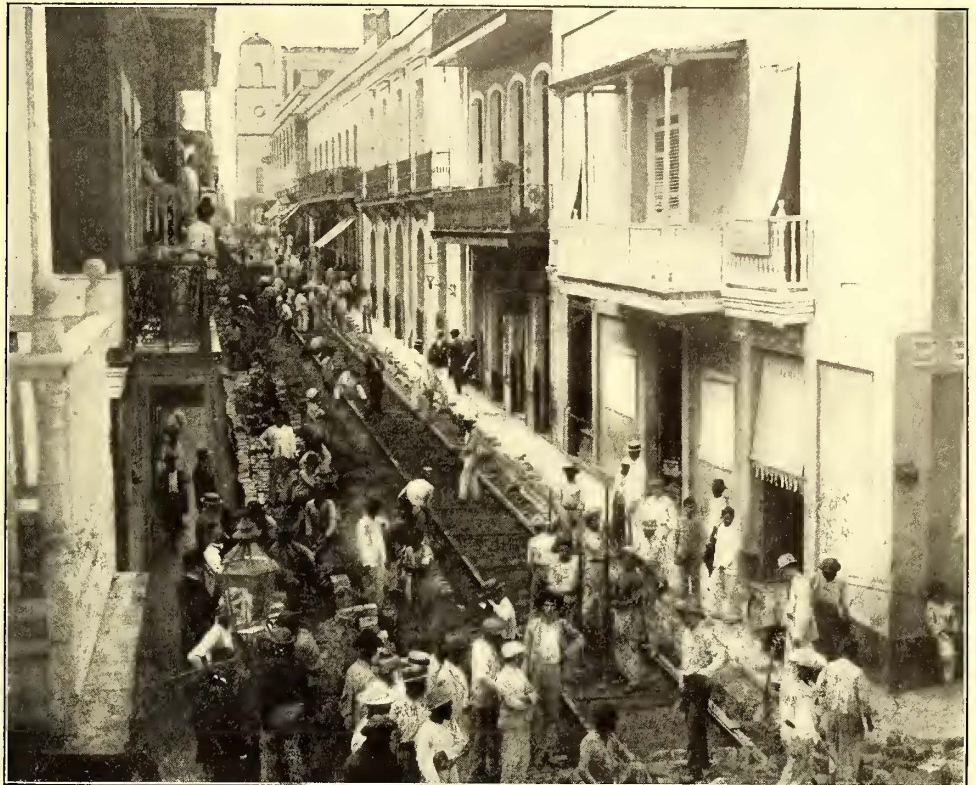
LAYING TRACKS IN SAN FRANCISCO STREET, A TYPICAL THOROUGHFARE IN SAN JUAN
