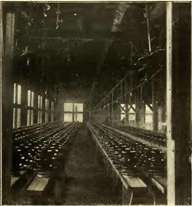
TESTING RACK FOR INSULATORS
