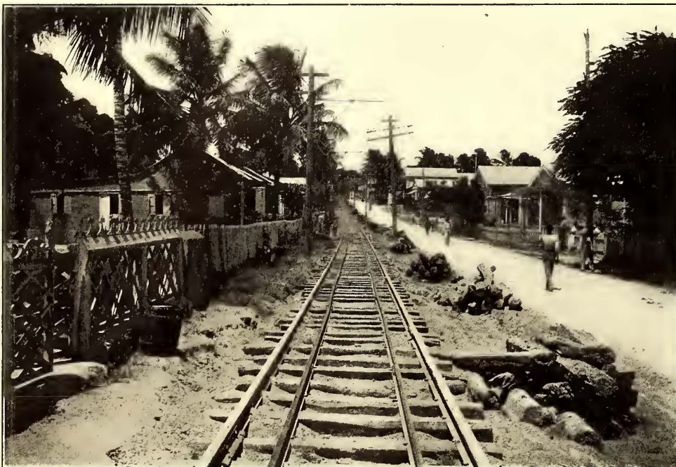
TRACK CONSTRUCTION ON THE CARATARA, SAN JUAN
