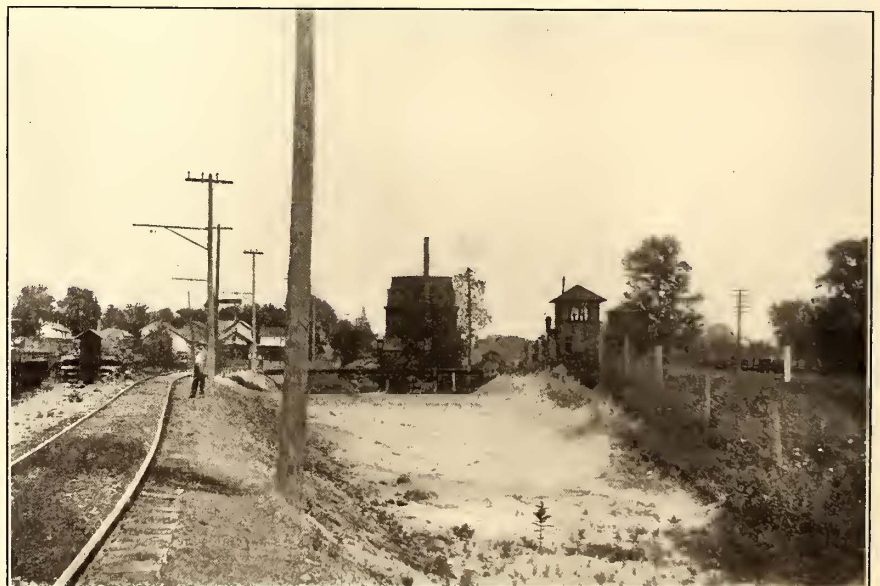
INTERLOCK AT WAUSEON, OHIO, PROTECTING TRACKS OF THREE ROADS—LAKE SHORE, DETROIT SOUTHERN AND THE TOLEDO & INDIANA RAILWAY
