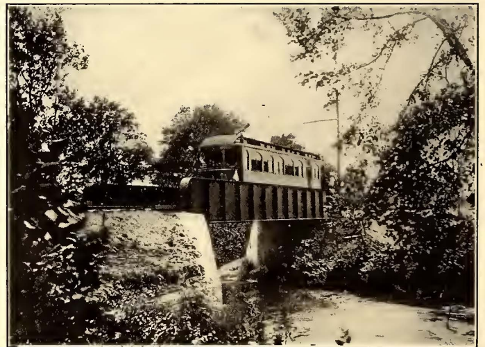
65-FT. THROUGH GIRDER BRIDGE ACROSS BEAVER CREEK, NEAR BRYAN, OHIO, ON THE LINE OF THE TOLEDO & INDIANA RAILWAY
