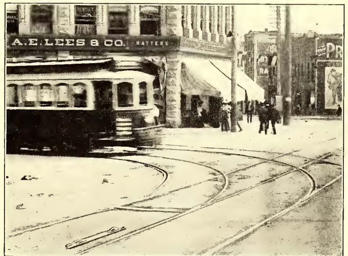
CAR APPROACHING A SWITCH
