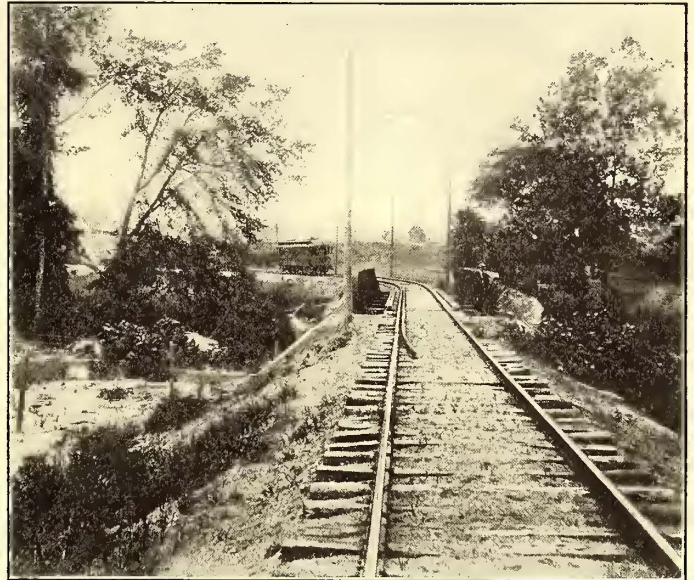
BEAVER CREEK BRIDGE AND UNDER CROSSING OF LAKE SHORE ON THE LEFT
