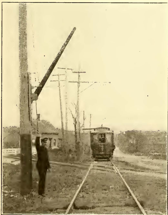
FIG. 1.—CONDUCTOR RAISING THE STOP-GATE
