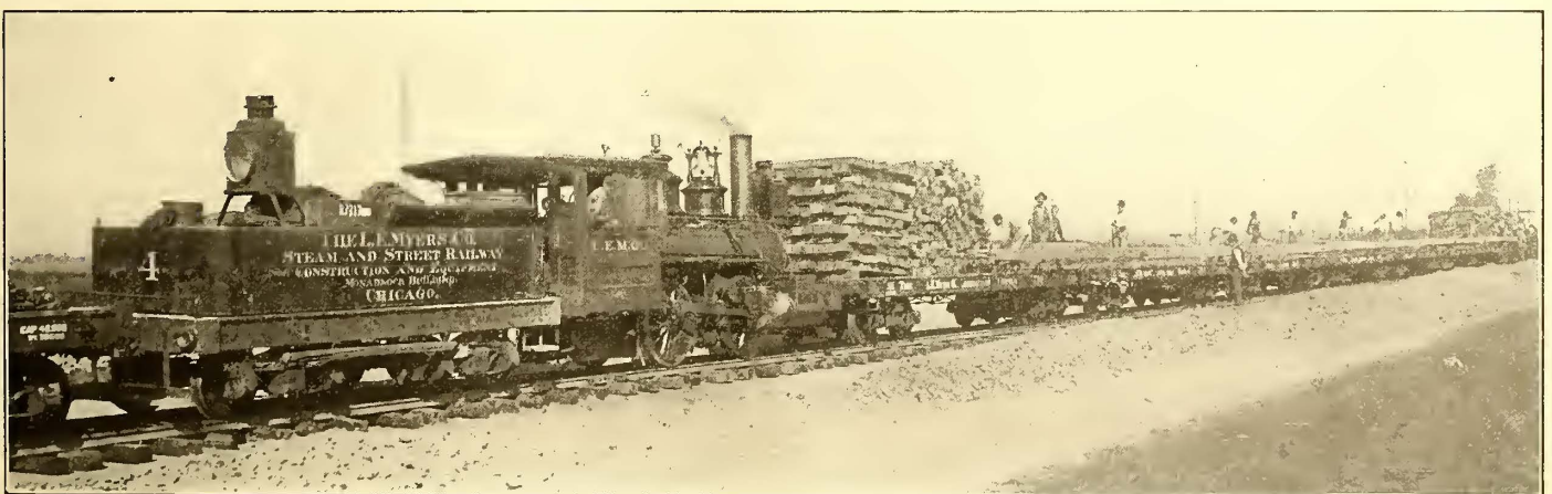
FIG. 3.—TRAIN OF CARS USED FOR THE TRACK-LAYING OPERATIONS ON THE FORT WAYNE & WABASH VALLEY TRACTION COMPANY
