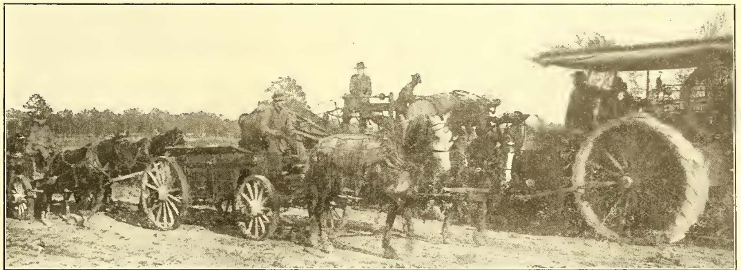
FIG. 2.—STEAM GRADER AT WORK ON THE LINE OF THE FORT WAYNE & WABASH VALLEY TRACTION COMPANY
