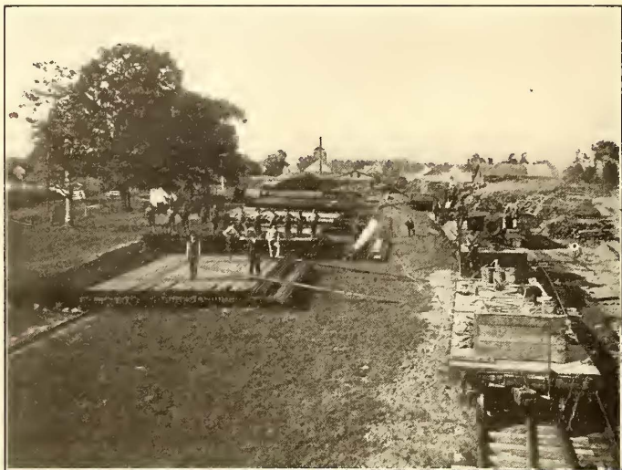
FIG. 5.—STORAGE YARD FOR TIES AND RAILS, USED IN THE BUILDING OF THE FORT WAYNE & WABASH VALLEY RY.
