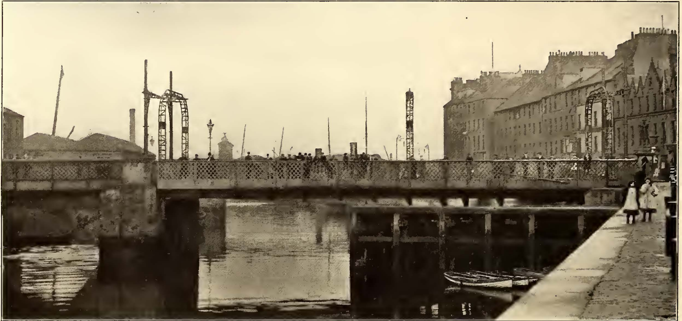
SWING BRIDGE ON BERNARD STREET, SHOWING METHOD OF MAKING CONNECTIONS
