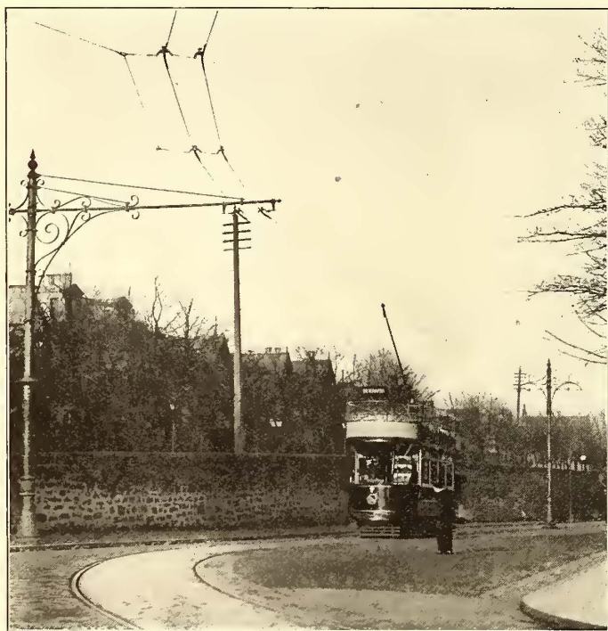
VIEW ON CRAIGHALL ROAD, SHOWING CURVE AND CENTER POLE CONSTRUCTION
