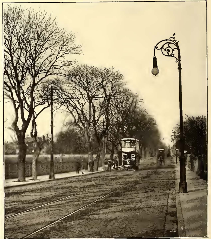
VIEW ON NEWHAVEN ROAD, SHOWING SIDE BRACKET POLE CONSTRUCTION
