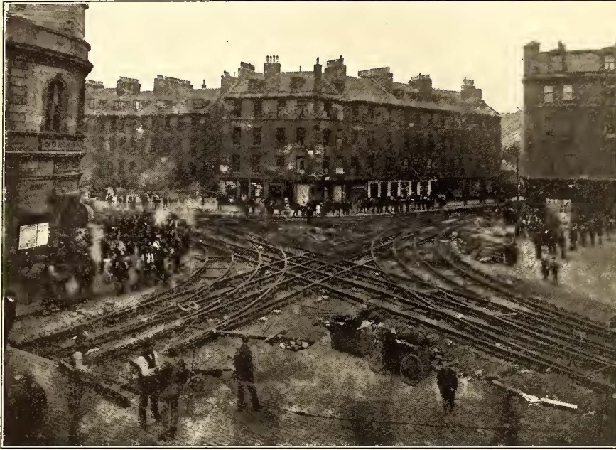
LARGE PIECE OF SPECIAL WORK IN LEITH
