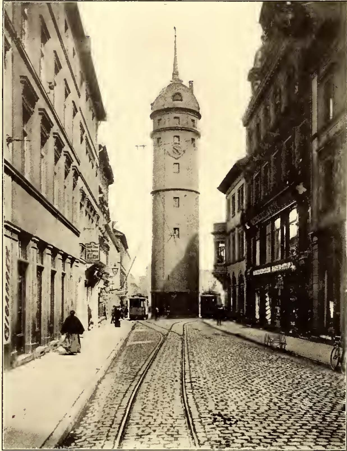
STREET IN DARMSTADT, SHOWING METHOD OF ATTACHING TROLLEY WIRES TO BUILDINGS
