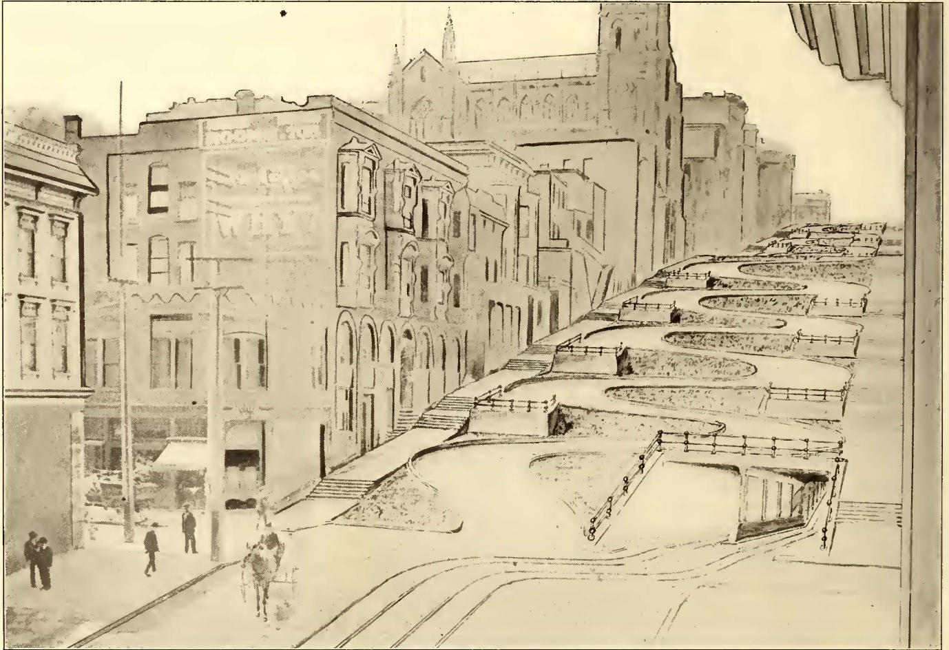
PERSPECTIVE PLAN, SHOWING SUGGESTION FOR TERRACING ROADWAY IN HILL DISTRICT, SAN FRANCISCO
