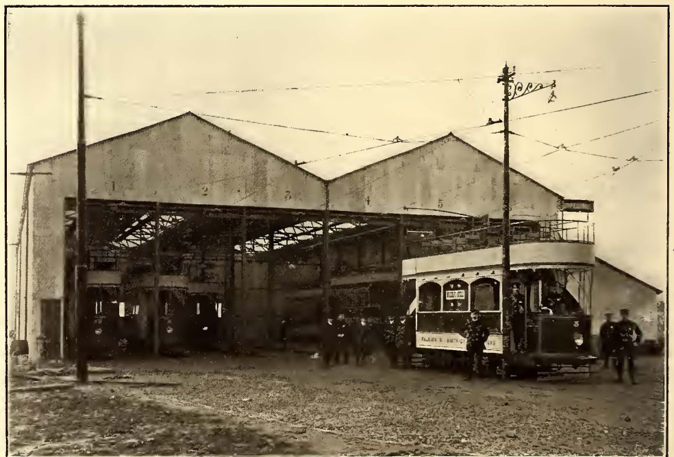
CAR HOUSE OF THE FALKIRK & DISTRICT TRAMWAYS, SHOWING IN PARTICULAR THE TYPE OF ROOF CONSTRUCTION
