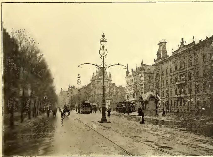
ORNAMENTAL CENTER-POLE CONSTRUCTION IN COLOGNE
