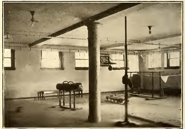
INTERIOR OF GYMNASIUM
