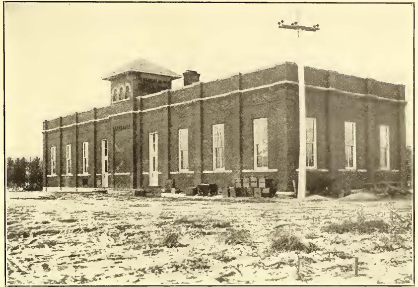
EXTERIOR OF NEW SUB-STATION
