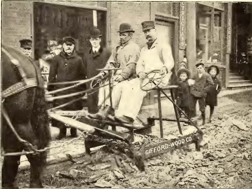
ICE-LEVELER IN SERVICE ON STREET
