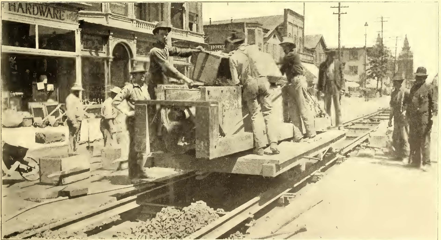
PORTABLE CONCRETE MIXER, SCRANTON RAILWAY
