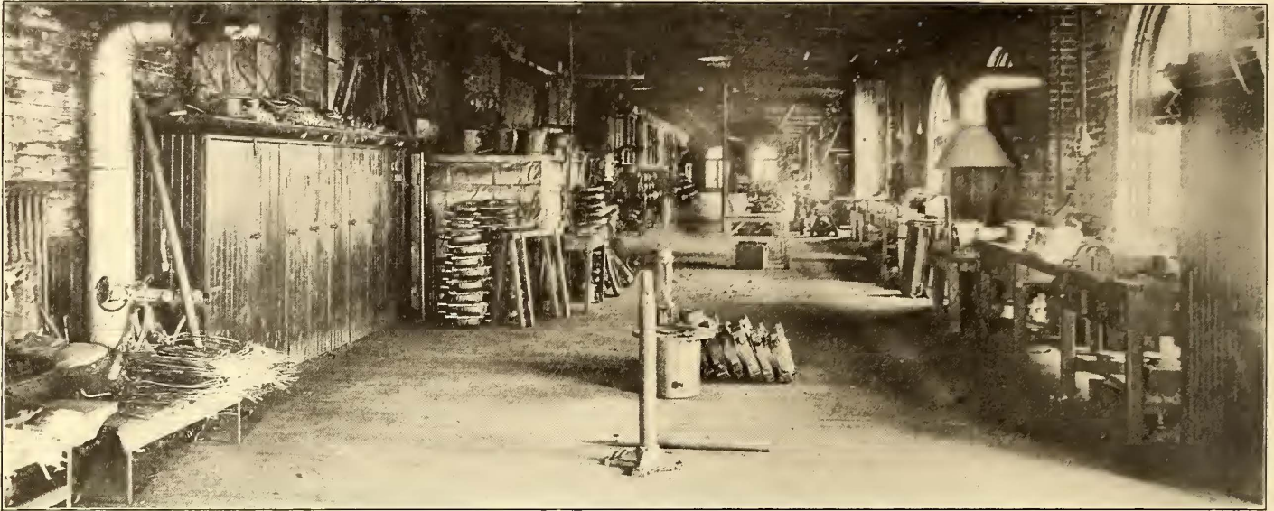
GENERAL VIEW OF FIELD AND ARMATURE ROOM, TORONTO RAILWAY SHOPS
