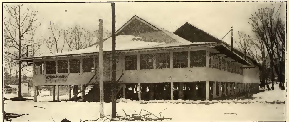
A VIEW OF THE EXTERIOR OF THE SKATING RINK IN BUSHKILL PARK
