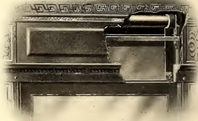
CUT-AWAY VIEW, SHOWING SASH BALANCE
