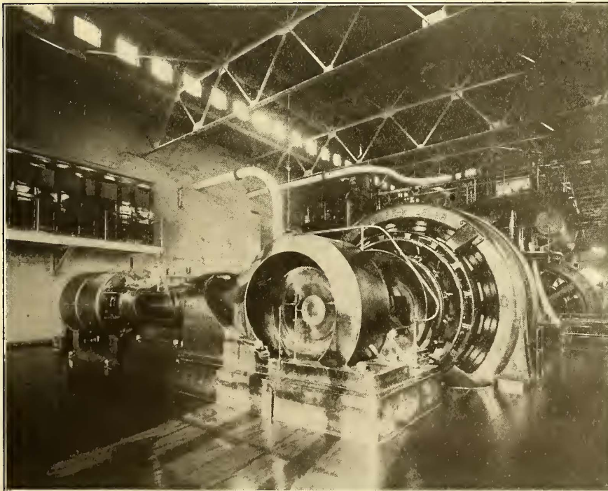
FIG. 4.—THE 900-KW GENERATING SET RECENTLY INSTALLED IN THE GRAND AVENUE POWER STATION, NEW HAVEN, CONN.
