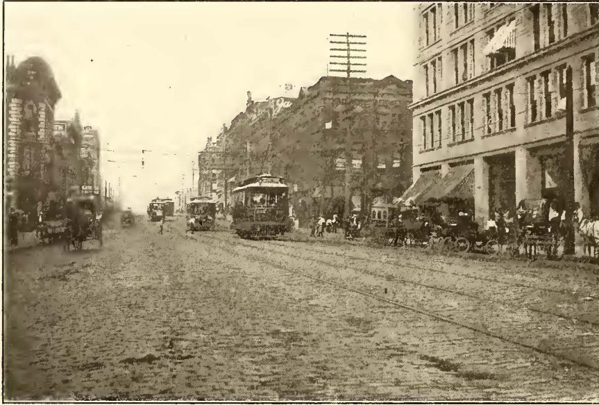
TYPICAL CONSTRUCTION ON PAVED STREETS IN BUSINESS DISTRICTS, BIRMINGHAM RAILWAY & ELECTRIC COMPANY
