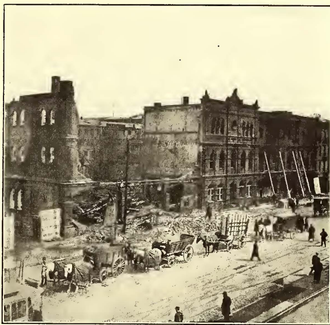
VIEW SHOWING ALL THAT REMAINED OF THE NEW YORK CITY RAILWAY CAR HOUSE AFTER THE FIRE, NAMELY, THE THREE-STORY OFFICE SECTION AND A PORTION OF THE WALLS
