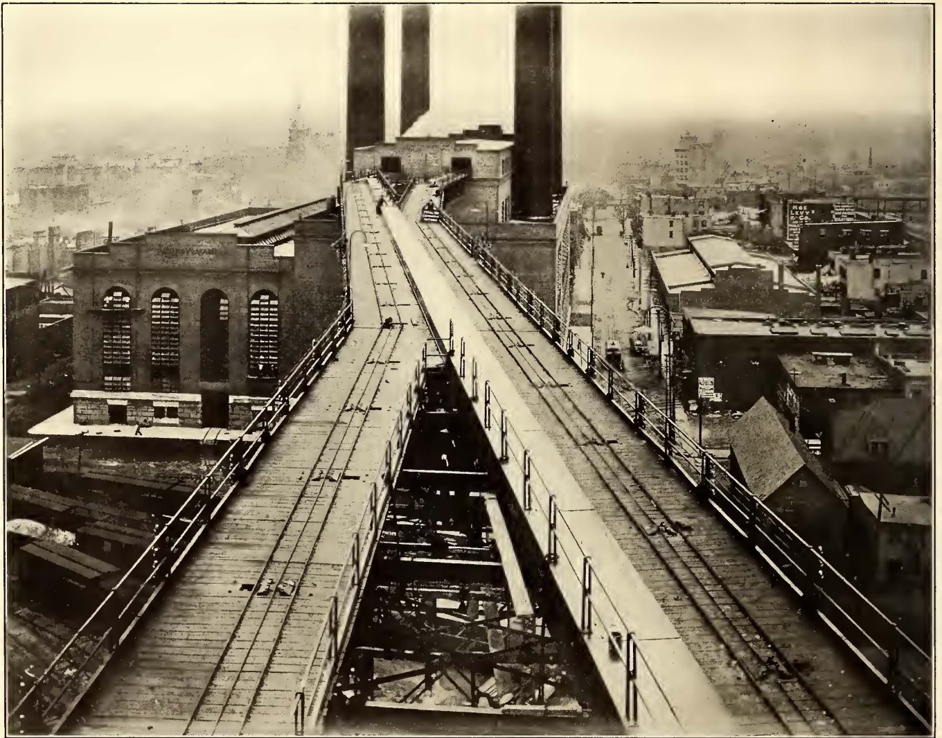
FIG. 3.—COAL BRIDGE, VIEWED FROM TOWER
