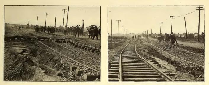
TWO SCENES ALONG THE LINES OF THE OAKLAND CONSOLIDATED TRACTION COMPANY, SHOWING THE UPHEAVAL OF THE ROADBED AND TWISTING AND BREAKING OF THE RAILS
