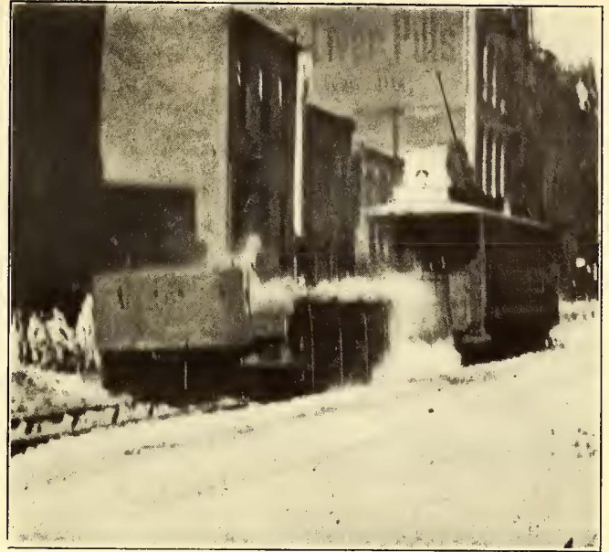
VIEW ON OLIVE STREET, TAKEN DURING EXPLOSION
