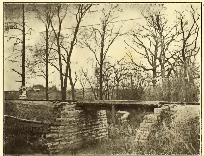
A 15-FT. SPAN WITH STONE BUTTRESSES
