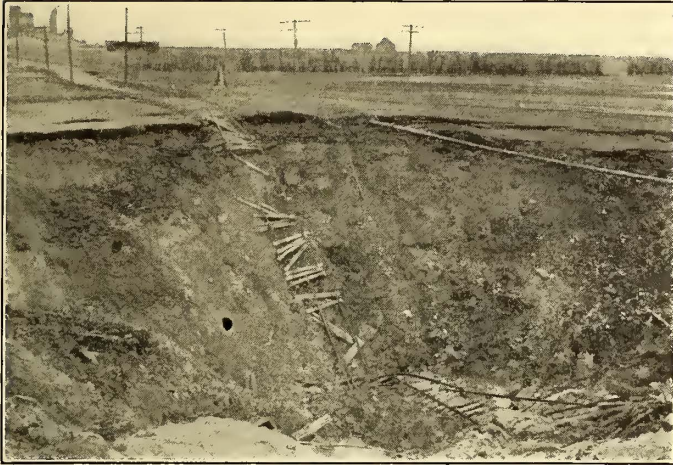
CAVE IN ON THE DUNENWEG LINE OF THE SOUTHWEST MISSOURI ELECTRIC RAILWAY COMPANY
