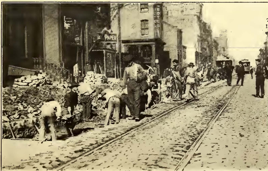
CLEARING AWAY THE DEBRIS AFTER AN EXPLOSION
