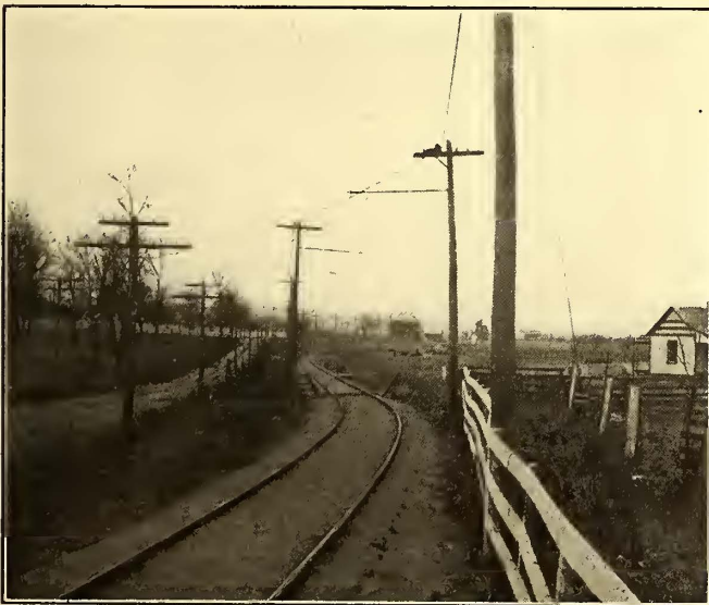
REVERSE CURVE BETWEEN FARMINGTON AND THE POWER HOUSE
