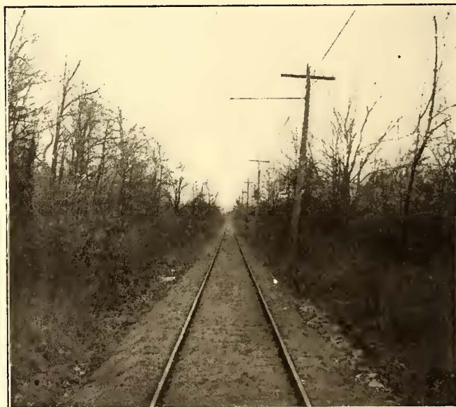
A TANGENT BETWEEN FARMINGTON AND FLAT RIVER, SHOWING HEAVY BALLAST
