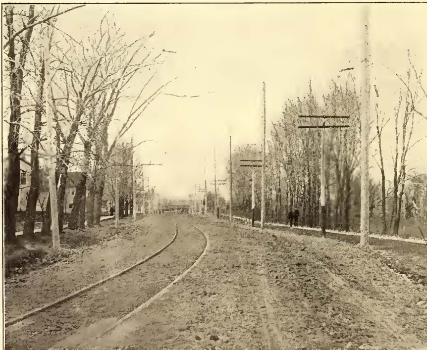
FIG. 3.—SPAN CONSTRUCTION WHERE BLOOMINGTON & PONTIAC LINE ENTERS DWIGHT
