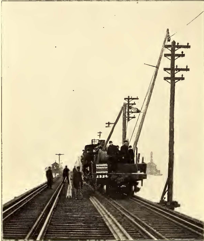
FIG. 18.—STRINGING CABLE ON JAMAICA BAY TRESTLE
