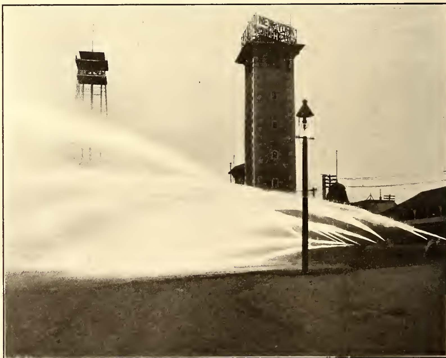
TEST OF HIGH-PRESSURE WATER SERVICE AT CONEY ISLAND, N. Y.
