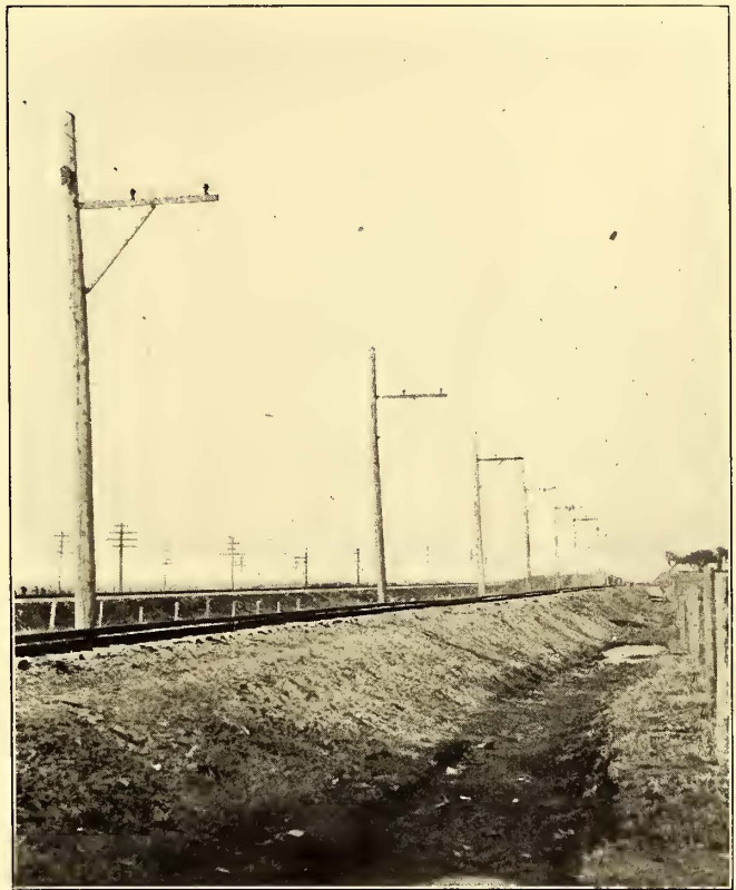
FIG. 1.—OVERHEAD CONSTRUCTION ON STRAIGHT TRACK
