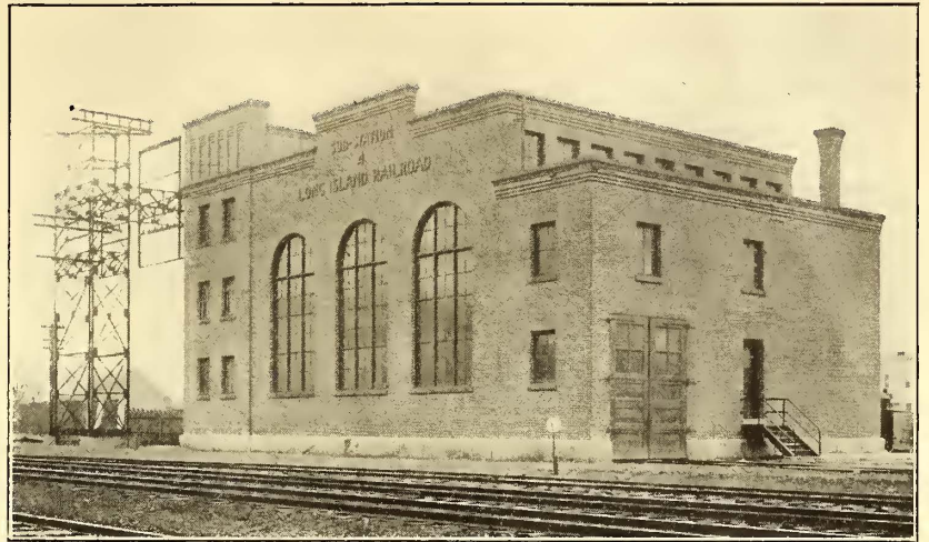
FIG. 9.—SUB-STATION AT ROCKAWAY JUNCTION
