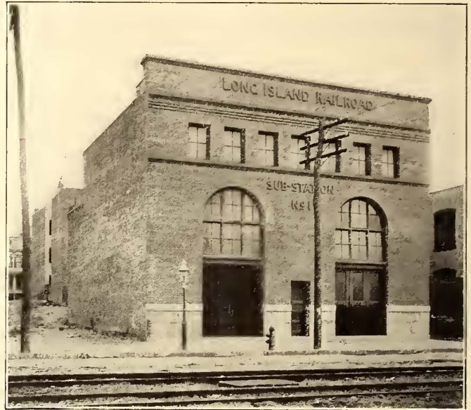
FIG. 4.—THE GRAND AVENUE SUB-STATION
