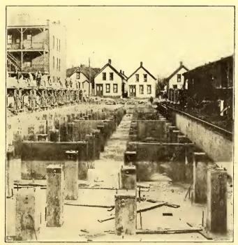
CONCRETE PIERS BEFORE THE RAILS, CHECKER-PLATES AND RADIATORS WERE INSTALLED
