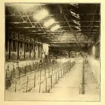
TWISTED RODS IN POSITION FOR CONCRETING TO FORM THE PIT PIERS
