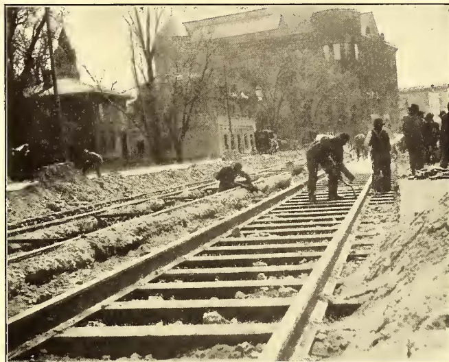
NEW TRACK CONSTRUCTION ON HENNEPIN AVENUE, MINNEAPOLIS
