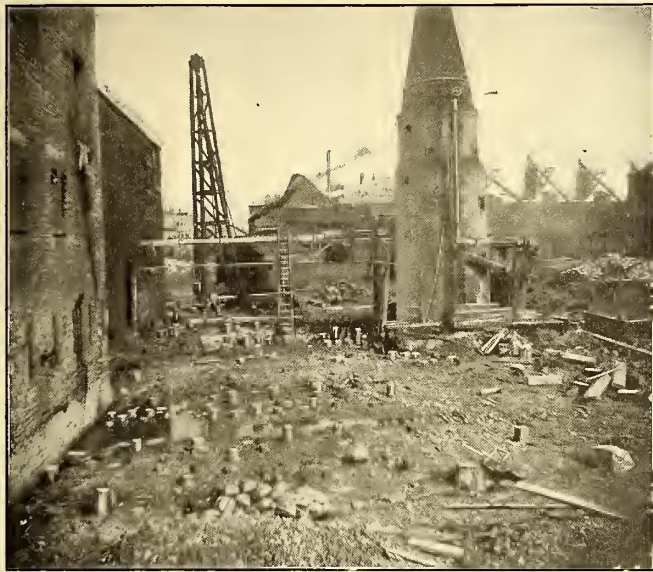
VIEW SHOWING THE PILING FOR THE SOUTH HALF OF THE PLANT, AND THE PORCUPINE BOILER SUPPLYING STEAM TO ENGINES IN THE BUILDING WHICH OCCUPIED THE SITE OF THE NORTH HALF OF THE PLANT
