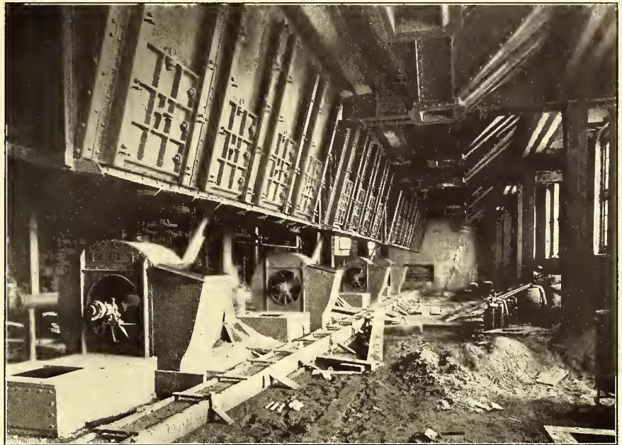
CONSTRUCTION VIEW OF PASSAGE-WAY UNDER THE BOILERS
