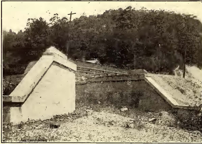
PLATE GIRDER BRIDGE WITH CONCRETE ABUTMENTS
