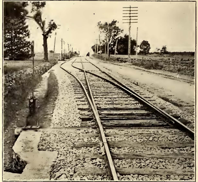
TYPICAL CONSTRUCTION AT A TURNOUT
