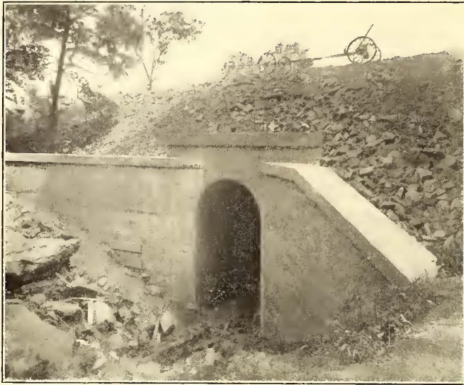
TYPICAL CONCRETE CULVERT
