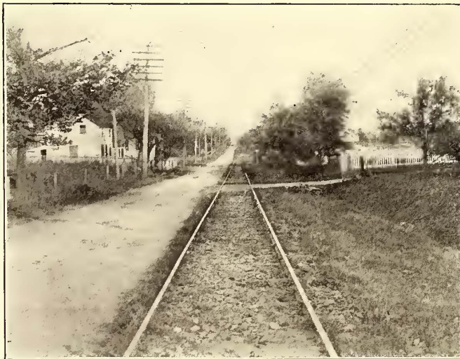
THE METAMORPHOSIS OF AN ELECTRIC RAILWAY. THE VIEW AT THE LEFT SHOWS THE OLD TRACK OF THE PHILADELPHIA & WEST CHESTER STREET RAILWAY, WITH UNCERTAIN SURFACING AND ALIGNMENT, SCANTY BALLAST AND ABUNDANT WEEDS ON THE ROADBED. THE VIEW ON THE RIGHT SHOWS THE PRESENT ROCK-BALLASTED TRACK
