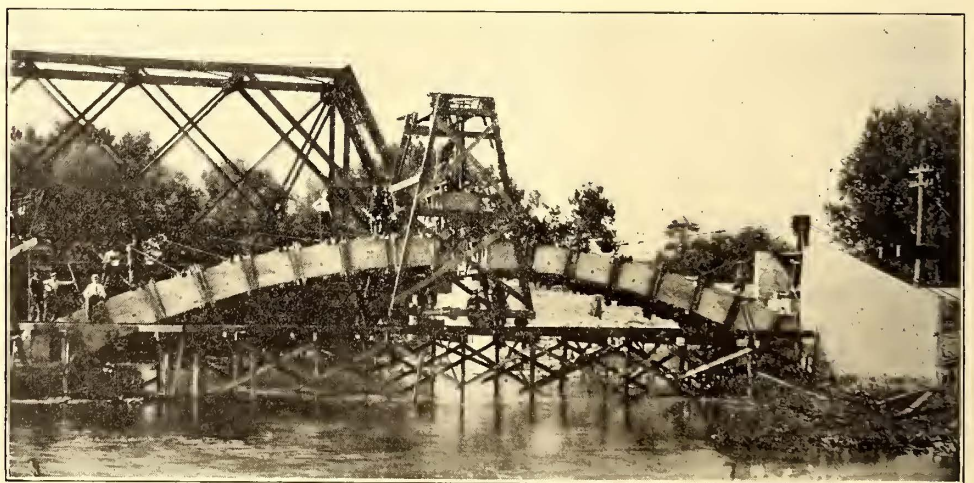
PLACING KEYSTONE IN ARCH
