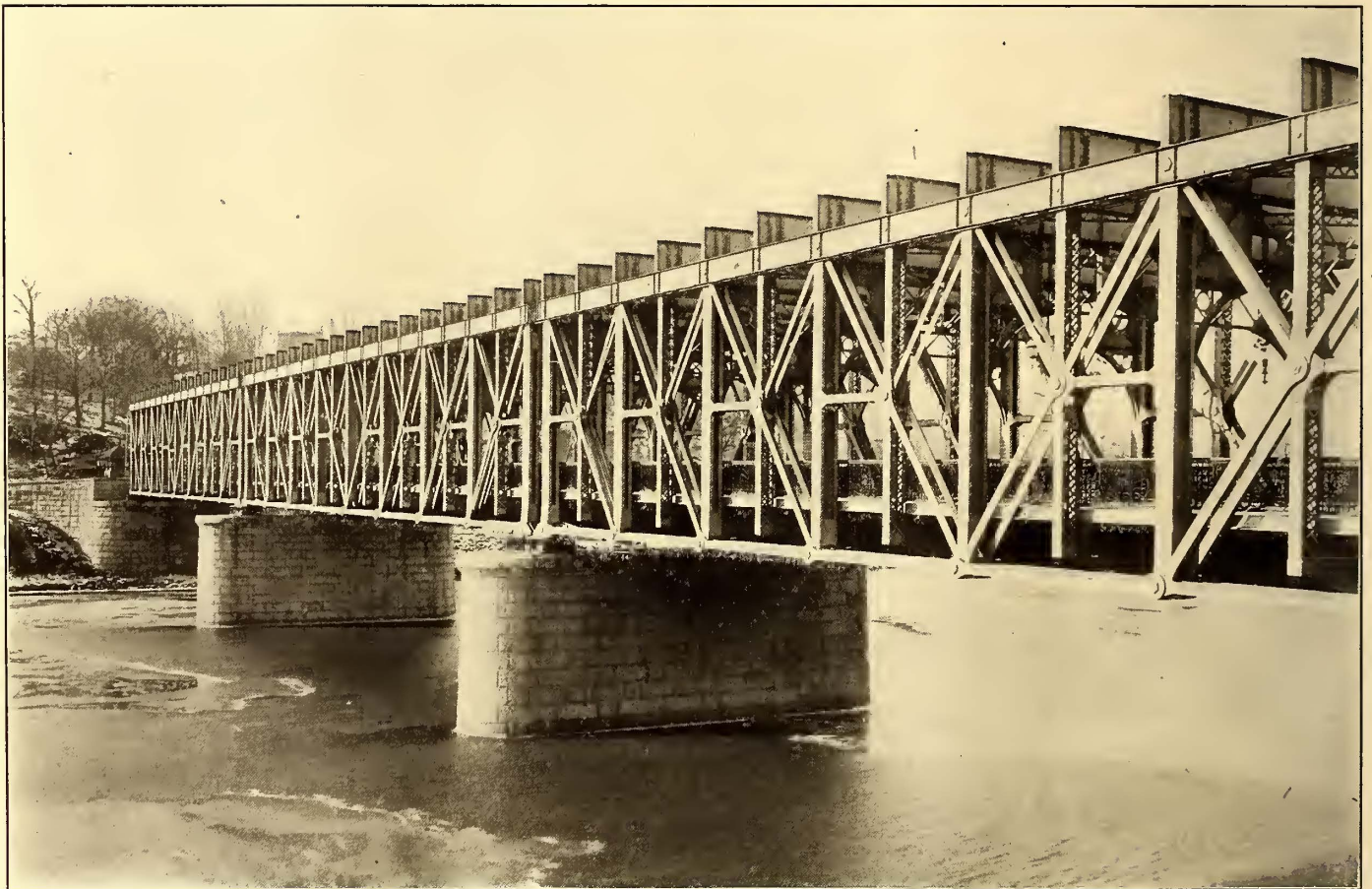
SCHUYLKILL RIVER BRIDGE AT FALLS OF SCHUYLKILL, PHILADELPHIA, PA.
