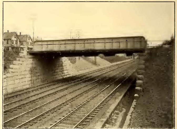
RICHARDSON STREET BRIDGE, NEWTONVILLE, MASS.
