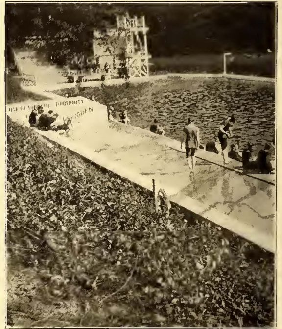
CONCRETE PLATFORM AND DIVING TOWERS, SWIMMING TANK, ROCK SPRINGS PARK
