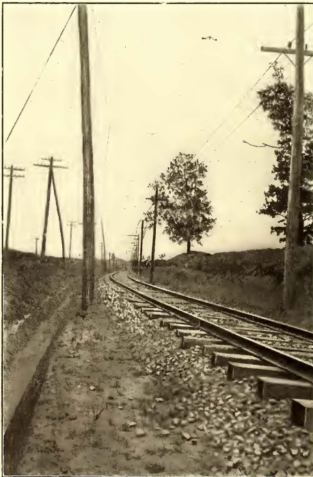
VIEW SHOWING DEPTH OF BALLAST AND TROLLEY CONSTRUCTION ON CURVES
