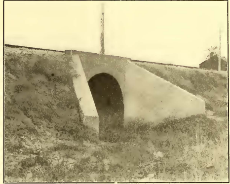
A 12-FT. CONCRETE CULVERT NEAR BLUFFTON
