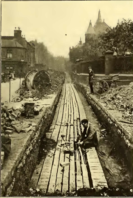
LAYING MAINS ON THE SOLID SYSTEM, BIRMINGHAM
