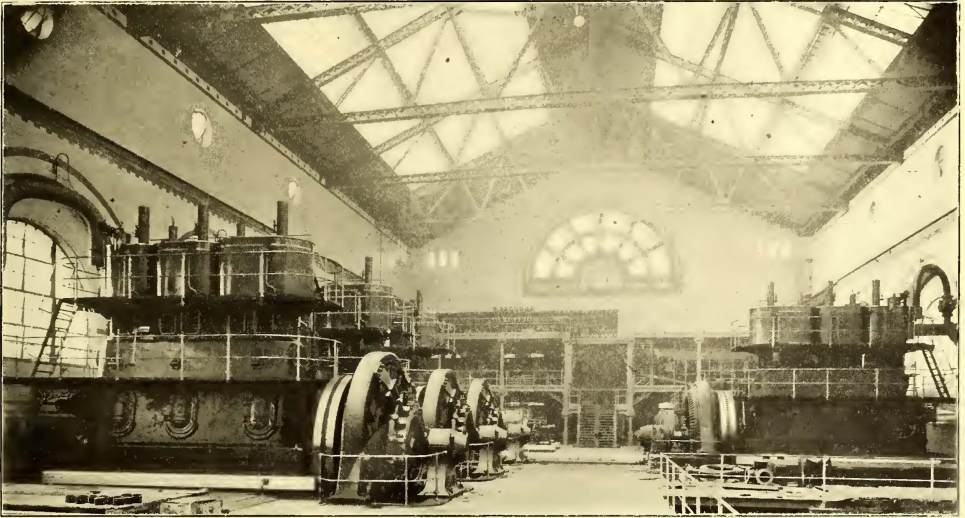
ENGINE ROOM, BIRMINGHAM
