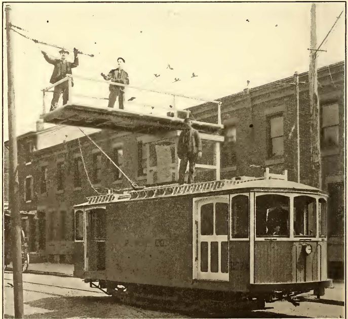
PHILADELPHIA TOWER CAR IN SERVICE, SHOWING EXTENSION PLATFORM
