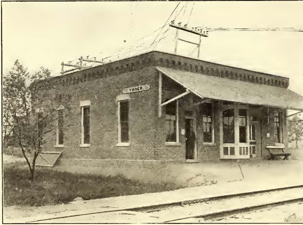
FREIGHT AND TICKET OFFICE SUB-STATION AT YODER
