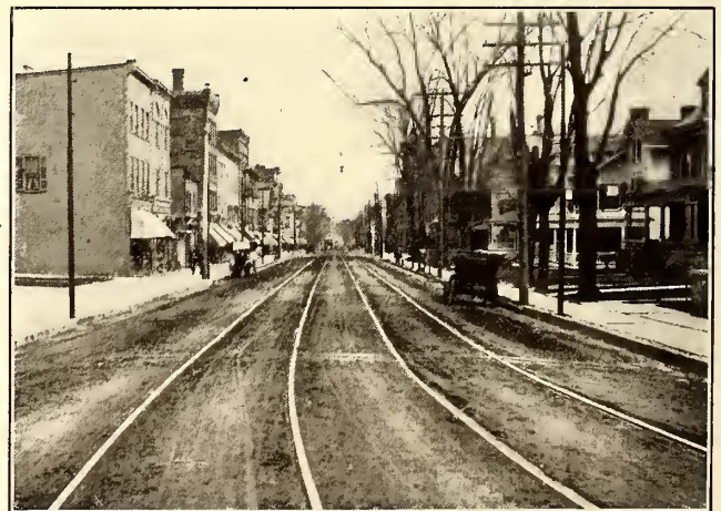
DOUBLE-TRACK PART OF THE LINE IN DOVER
