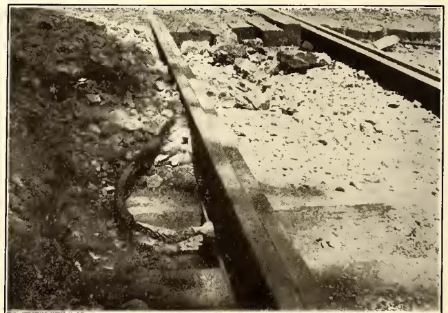
JOINT WELD WITH CABLE BOND
