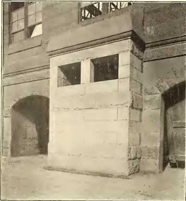
SIDE VENTILATOR AT BROAD STREET STATION
