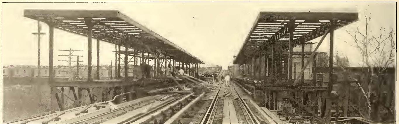
AT MARKET AND SIXTY-THIRD STREETS, WHERE THE THIRD RAIL IS PLACED BETWEEN THE TRACKS
