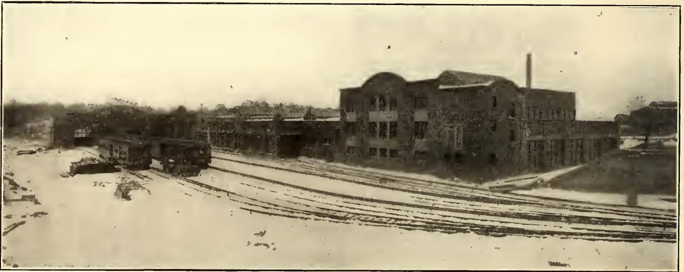
INSPECTION AND SHOP BUILDINGS OF THE PHILADELPHIA RAPID TRANSIT COMPANY, NEAR THE MARKET STREET TERMINAL
