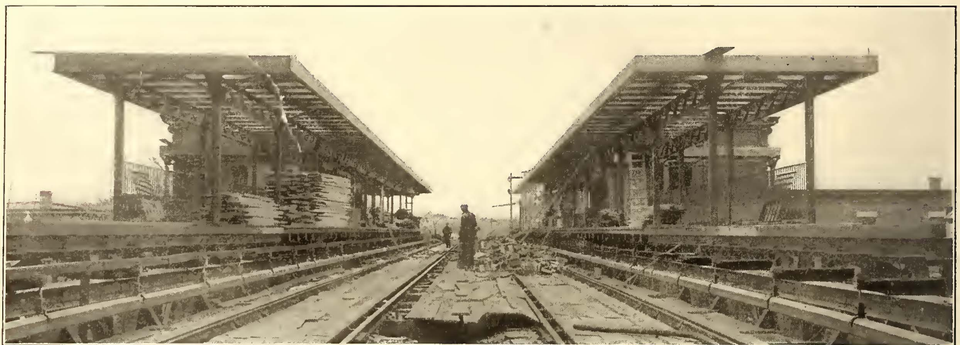
VIEW SHOWING METHOD OF THIRD-RAIL SUSPENSION ADOPTED ON THE MARKET STREET ELEVATED LINE TO SIXTY-THIRD STREET
