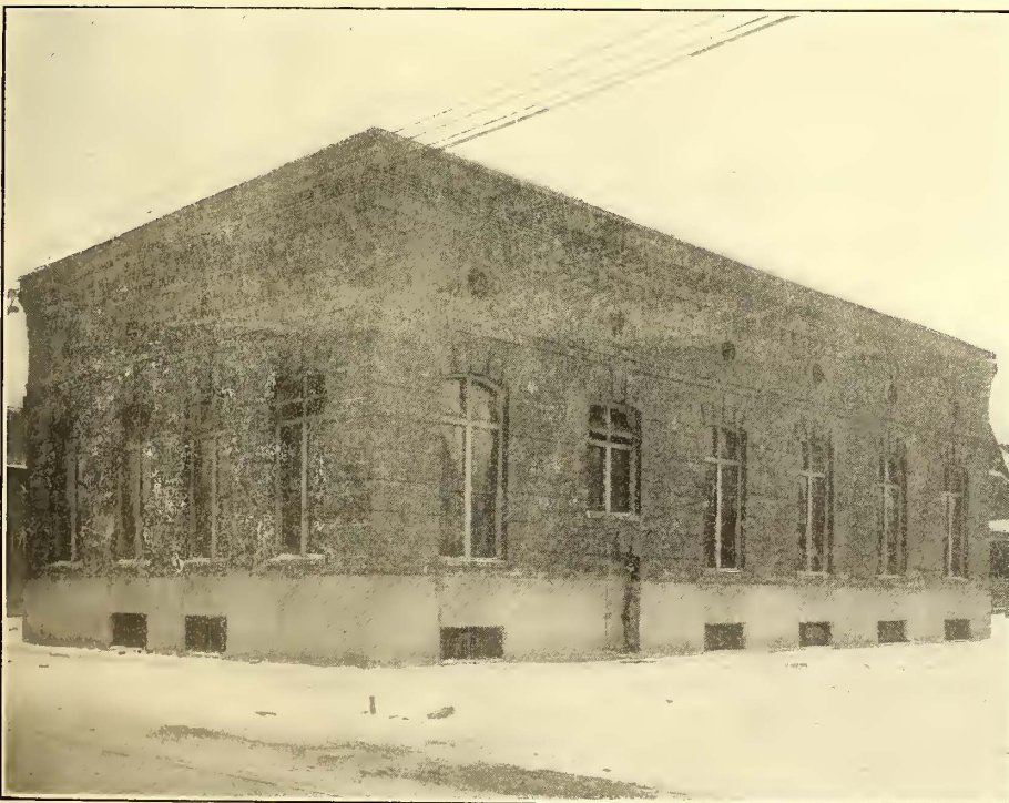
EXTERIOR VIEW OF THE SENECA STREET SUB-STATION OF THE INTERNATIONAL RAILWAY COMPANY, BUFFALO, N. Y.
