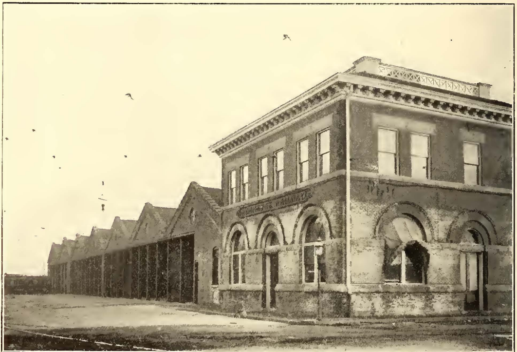
FRONT VIEW OF SHOPS AND OFFICE OF THE MEMPHIS STREET RAILWAY
