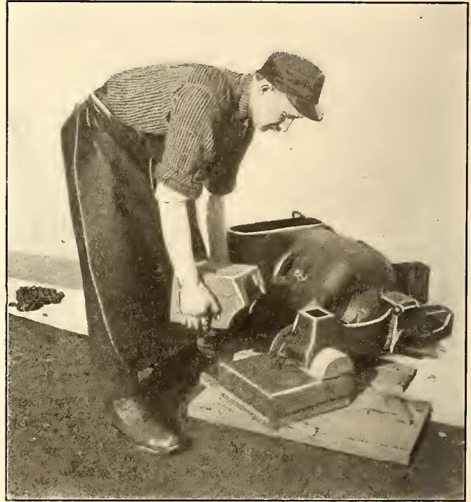
FIG. 3.—PLACING THE MOLD ON THE MOTOR BEFORE WELDING
