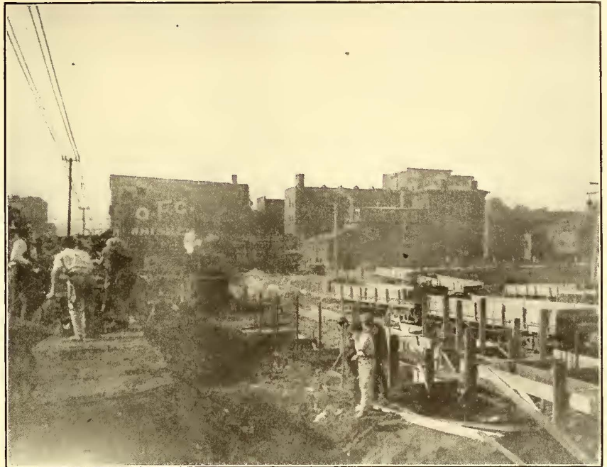
VIEW OF EXCAVATION, LOOKING WEST FROM SEVENTEENTH STREET
