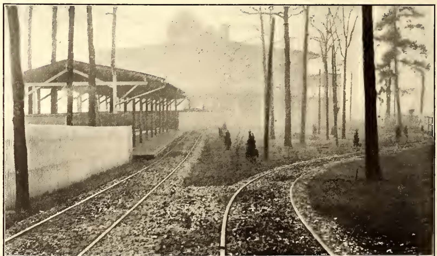
LOADING YARD AND LAY-OVER TRACK AT THE HOT SPRINGS RACE TRACK
