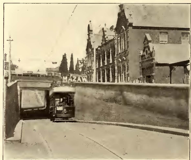
A VIEW IN THE OPEN CUT
