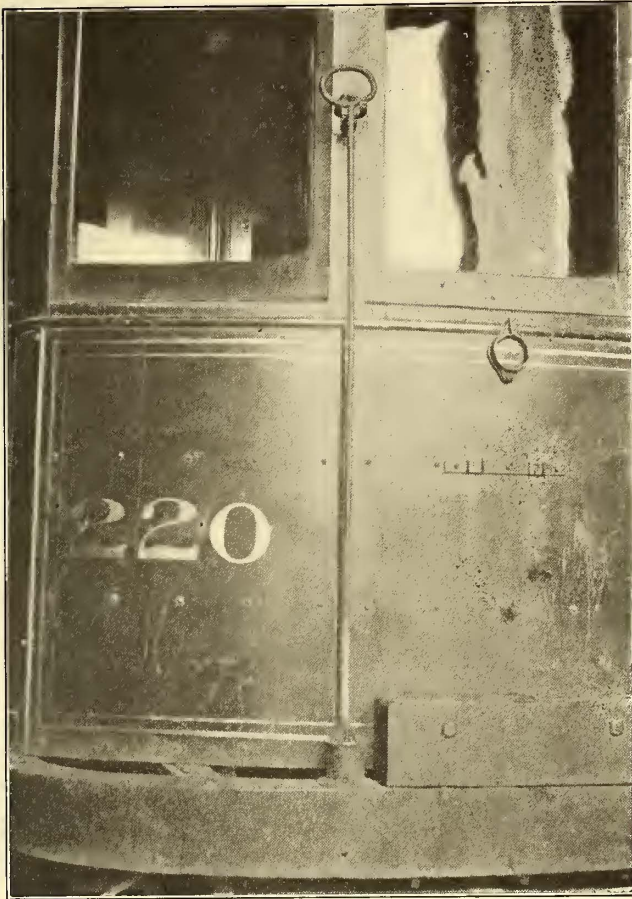
METHOD OF HANGING SWITCH-ROD AT LITTLE ROCK
