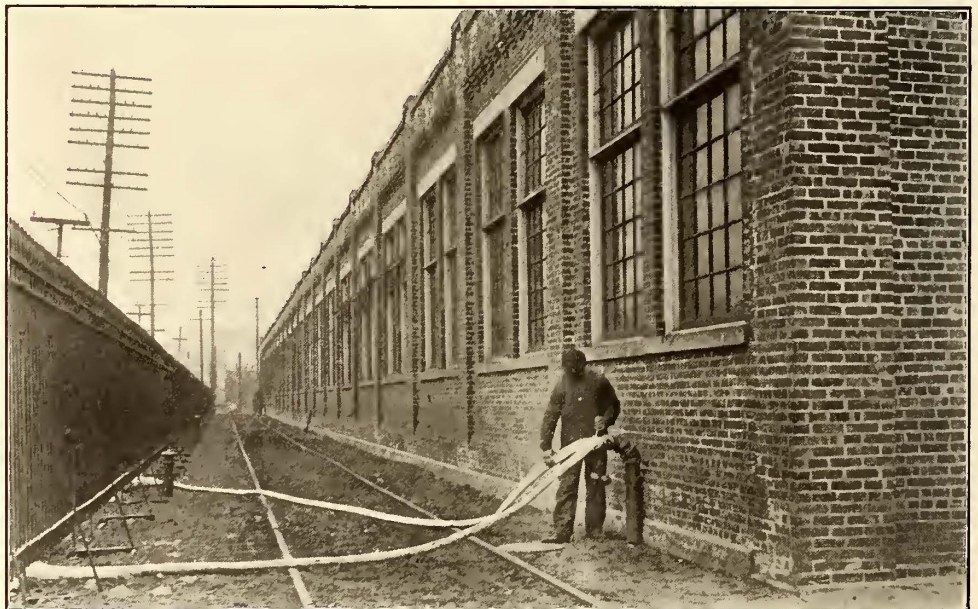
FIG. 18.—ONE OF THE HOSE CONNECTIONS ALONGSIDE THE SHOP BUILDING
