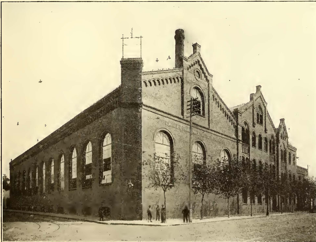
EXTERIOR VIEW OF THE THREE-PHASE STATION, CORNER MONTEVIDEO AND PASEO DE JULIO, OPERATED BY THE GERMAN TRANSATLANTIC ELECTRICITY COMPANY, BUENOS-AIRES
