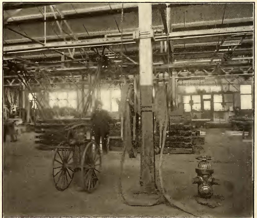
FIG. 9.—CHEMICAL ENGINE AND FIRE HYDRANTS IN THE PLANK ROAD SHOPS
