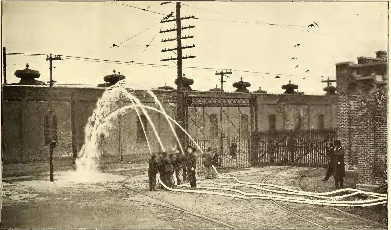
FIG. 14.—A VIEW OF THE FIRE-HOSE STREAMS WITH THE CITY PRESSURE OF ONLY 25 LBS.
