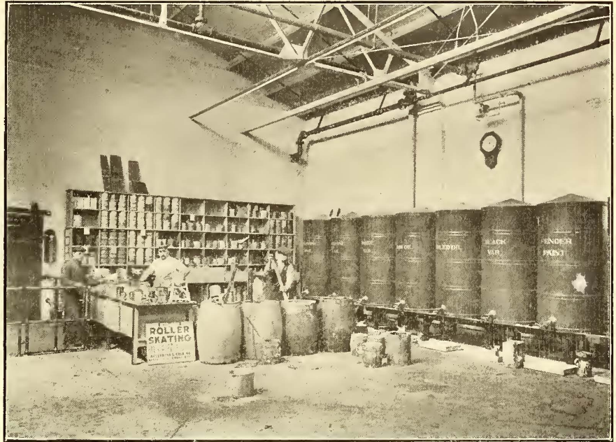
FIG. 3.—INTERIOR OF PAINT STOREROOM
