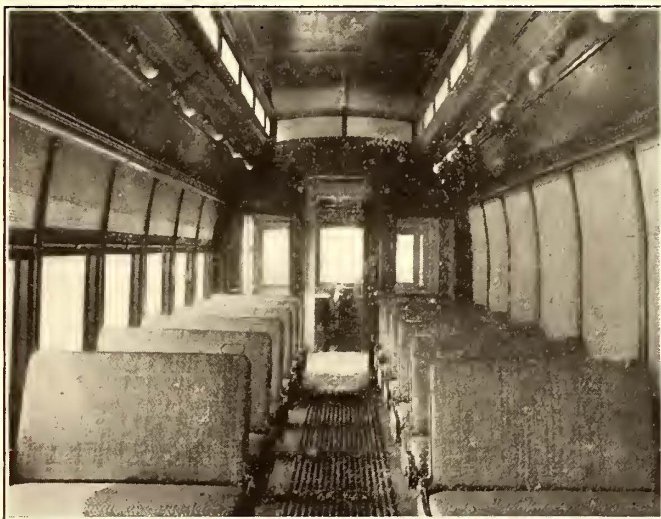
INTERIOR OF BOISE COMBINATION CAR, SHOWING SEATING AND LIGHTING ARRANGEMENTS
