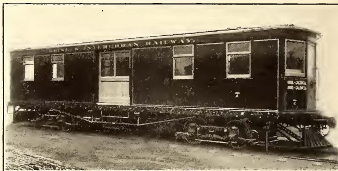
EXTERIOR OF BOISE FREIGHT CAR
