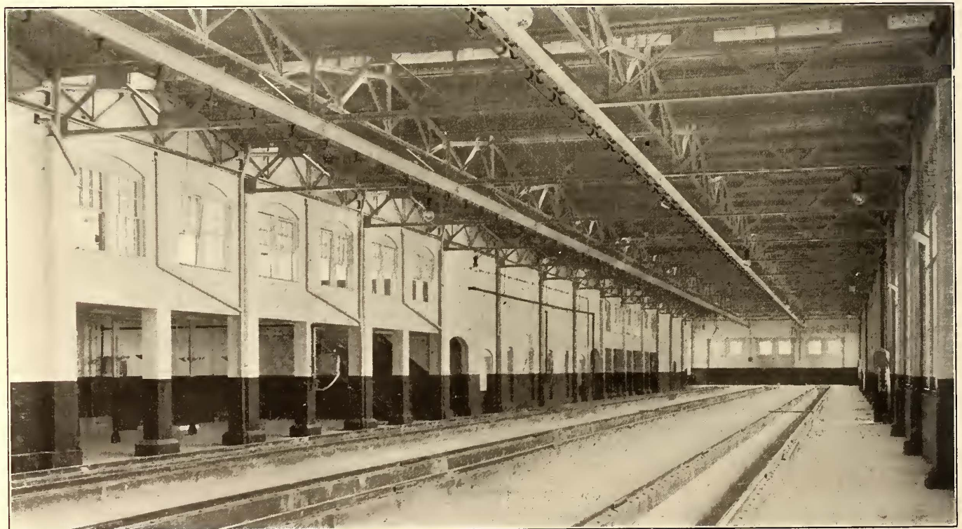
INTERIOR VIEW OF THE HARMON INSPECTION SHED, SHOWING THE POSITION OF THE FACILITIES ROOMS
