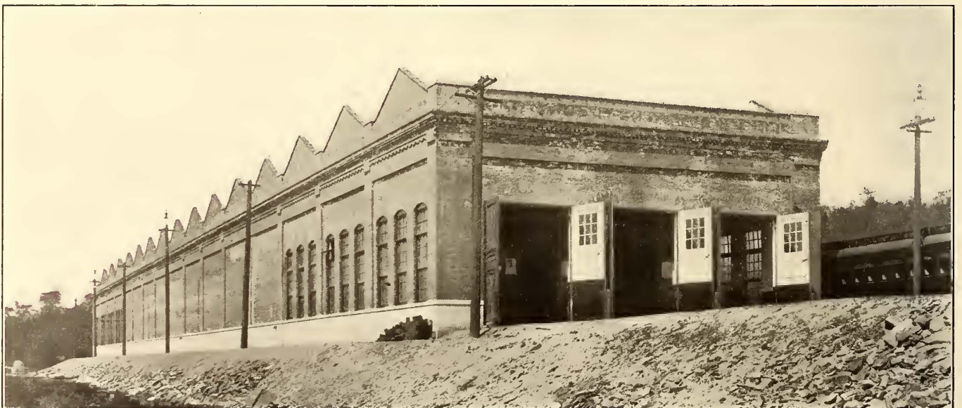
ENTRANCE TO THE NORTH WHITE PLAINS INSPECTION BUILDING
