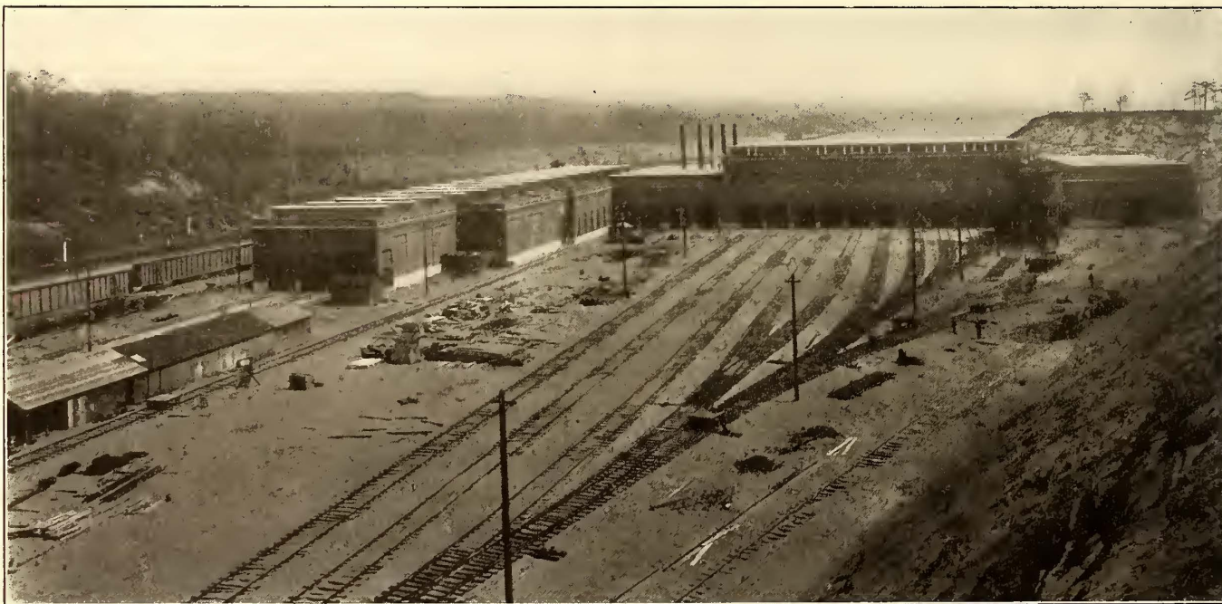
GENERAL VIEW OF THE HARMON SHOPS, LOOKING SOUTH
