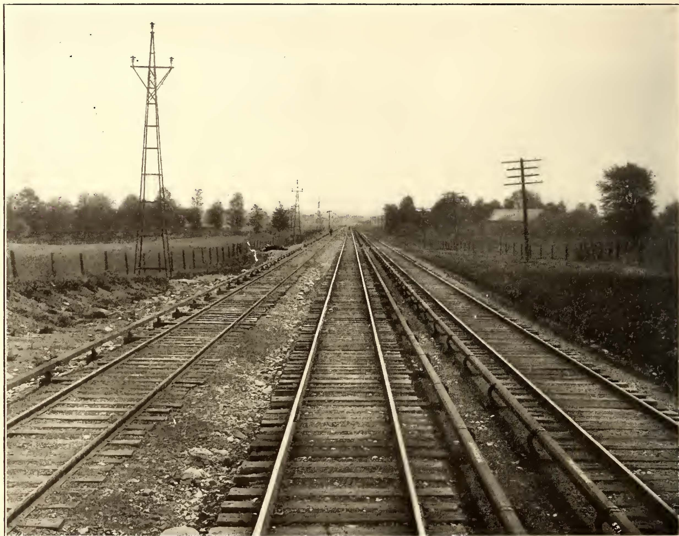
TYPICAL CONSTRUCTION ON TANGENTS, LOOKING EAST ALONG A THREE-TRACK SECTION
