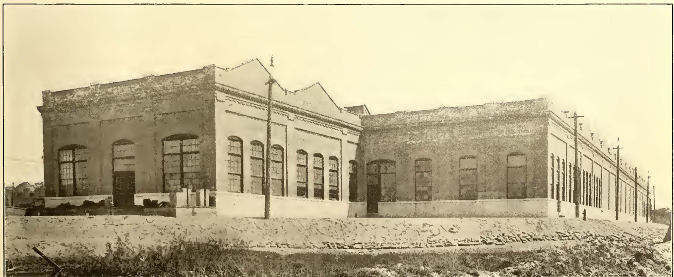
THE NORTH WHITE PLAINS PLANT, SHOWING THE POSITION OF THE FACILITIES ROOMS
