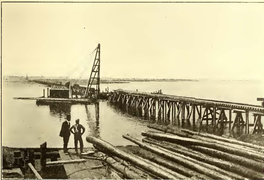
TRESTLE UNDER CONSTRUCTION ACROSS GREAT EGG HARBOR
