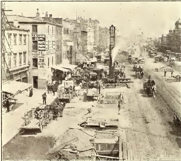
TWO VIEWS ALONG DELAWARE AVENUE, PHILADELPHIA, SHOWING THE FOUNDATIONS OF ELEVATED PILLARS
