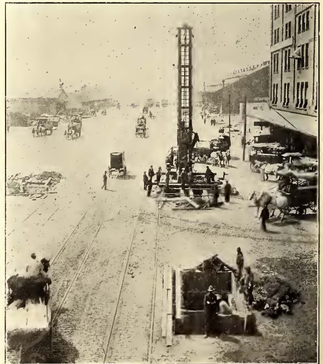
TWO VIEWS ALONG DELAWARE AVENUE, PHILADELPHIA, SHOWING THE FOUNDATIONS OF ELEVATED PILLARS
