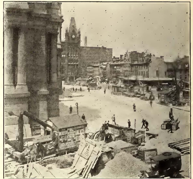
AT WORK ON THE LOOP AROUND THE CITY HALL
