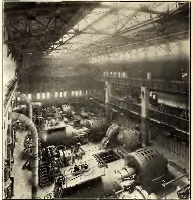
INTERIOR VIEW OF THE DELAWARE AVENUE STATION
