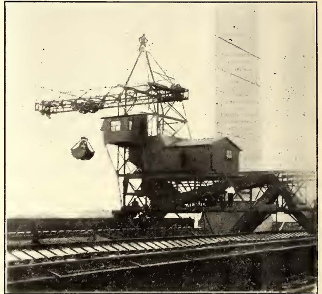
COAL-HANDLING APPARATUS AT THE NORFOLK POWER STATION
