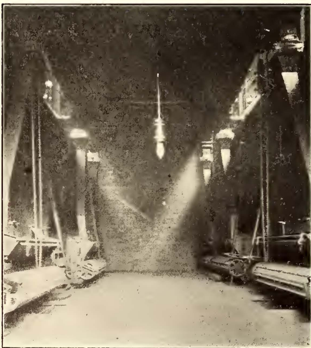
MECHANICAL STOKERS IN THE BOILER ROOM
